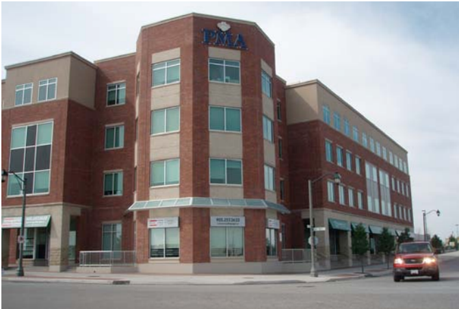
Image 8 - Oak Park Business Centre at Oak Park Boulevard and Taunton Road
