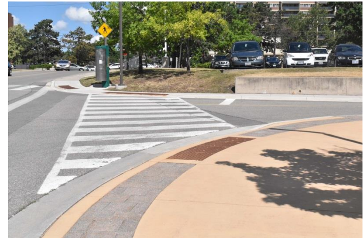
Curb ramps creating accessible exterior path of travel (3.1.20)
