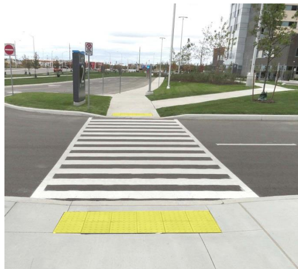
Well defined exterior path of travel (3.1.1)
