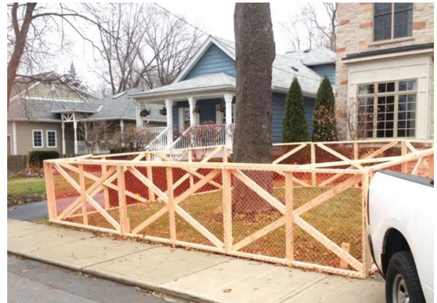
No disturbance of grade or storage of materials permitted within tree protection zones (2.3.6)
