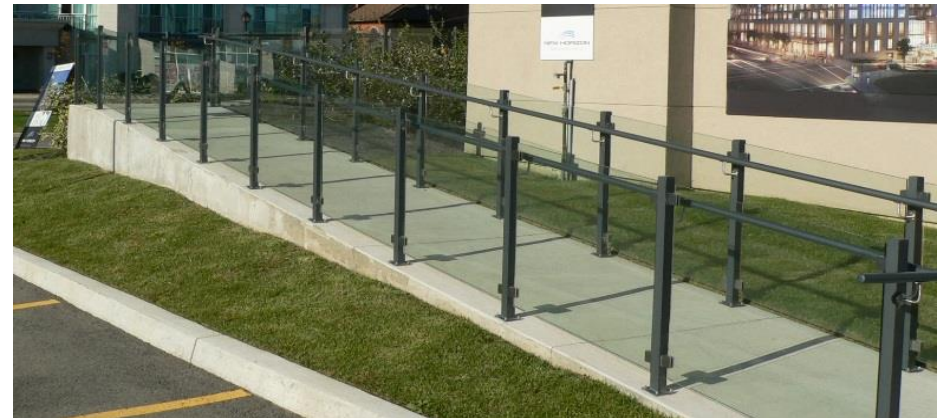
Barrier free ramp with hand rails and guards (3.1.15)
