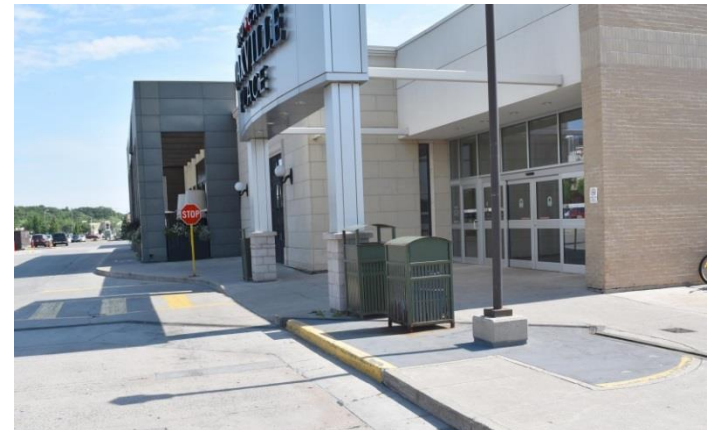
Pedestrian loading area located in close proximity to main entrance (3.2.17)
