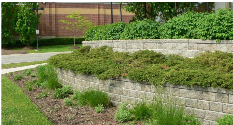
Terraced retaining walls providing appropriate transition in grade (2.4.4)
