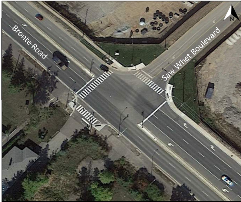
Figure 4: Saw Whet Boulevard at Bronte Road
