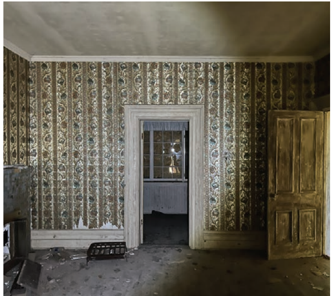
Looking towards the enclosed sunroom off of one of the two front rooms on the ground floor (ERA, 2025).
