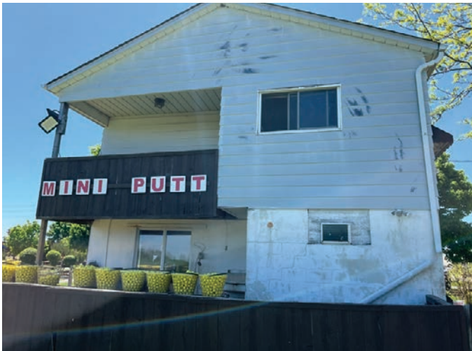
Side (east) elevation (ERA, 2025).
