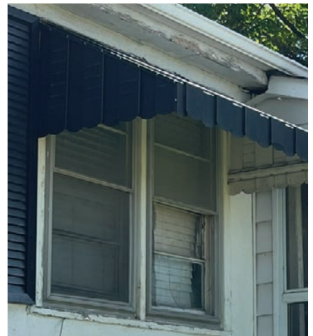
Metal windows in fair condition (ERA, 2025).
