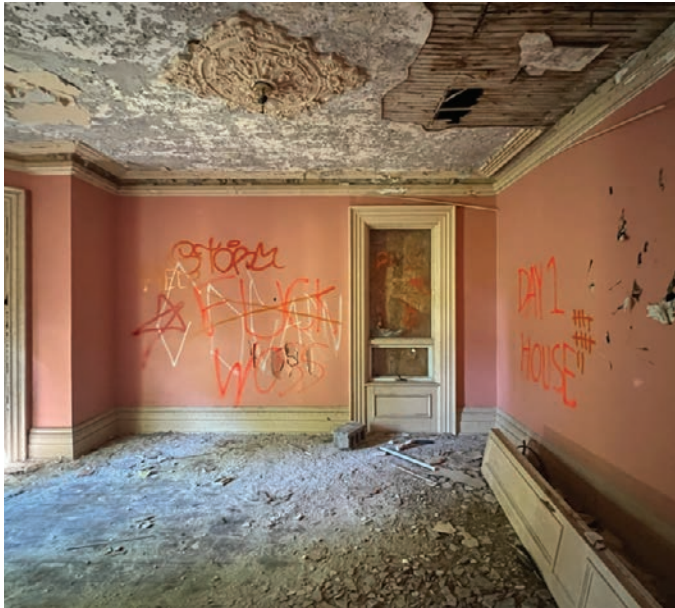
Looking into one of the two front rooms on the ground floor (ERA, 2025).
