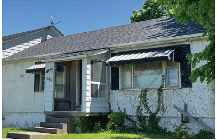
Asphalt roof shingles in good condition (ERA, 2025).
