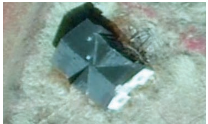
2006 close-up aerial photo of the farmhouse at 340 Burnhamthorpe Road East. Note the two openings on the east and south elevations where the fireplace and rear addition would have been prior to the relocation of the building (Town of Oakville).
