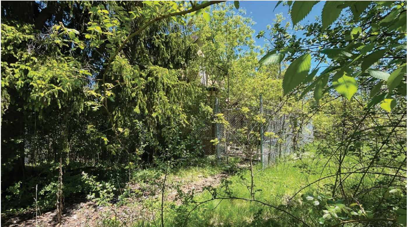
Looking southeastward towards the principal (west) elevation of the building at 3437 Trafalgar Road from behind the security fence (ERA, 2025).
