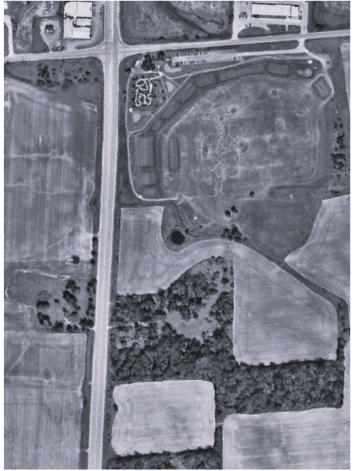
Circa 2024 aerial of the Site following the relocation of the mid-19th century dwelling at 340 Burnhamthorpe Road and widening of the intersection (Google).
