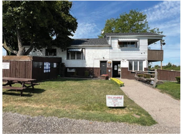
Rear (south) elevation of mid 20th-century house-form building at 340 Burnhamthorpe Road (ERA, 2025).
