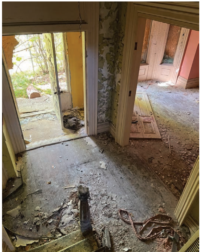
Looking down into the hallway on the ground floor from the staircase (ERA, 2025).
