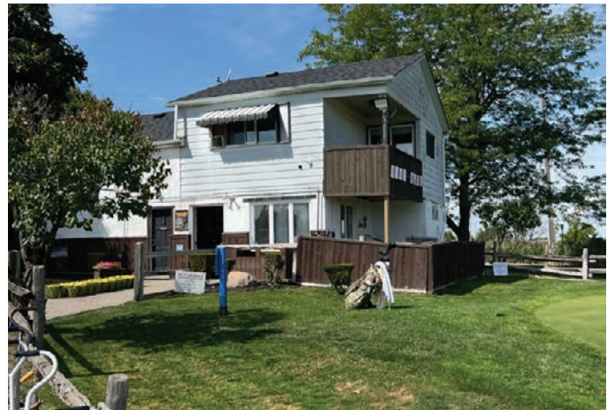
Rear (south) and side (east) elevations (ERA, 2025).
