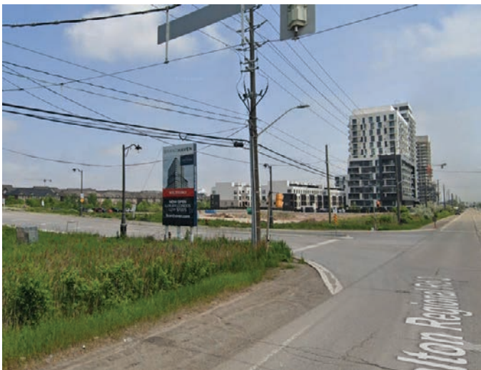
Looking southeast from the intersection of Trafalgar Road and Threshing Mill Boulevard, where residential construction is ongoing (Google, 2025).
