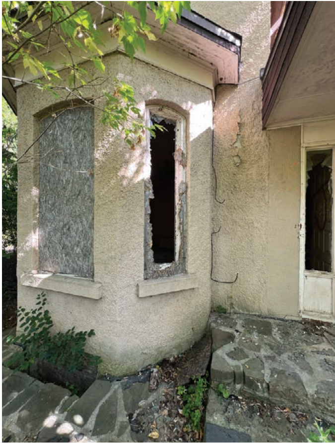
Bay window at the principal (west) elevation (ERA, 2025).
