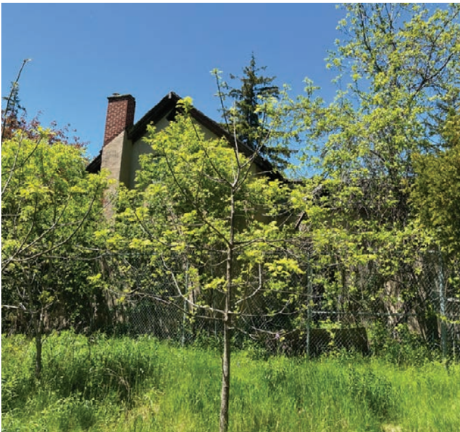
Looking towards the south elevation of the building at 3437 Trafalgar Road from behind the security fence (ERA, 2025).
