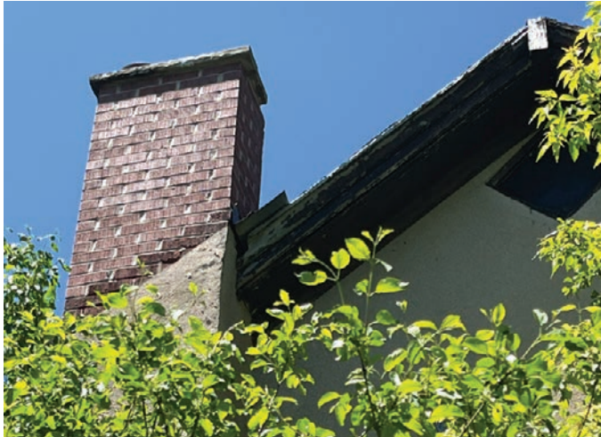
Exposed brick chimney at the roofline in fair condition (ERA, 2025).
