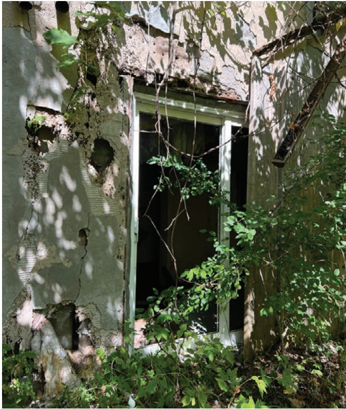
Looking towards the pair of sliding doors on the south elevation, leading into the kitchen (ERA, 2025).
