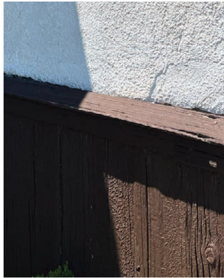
Wood siding in fair condition, with areas of poor condition (ERA, 2025).
