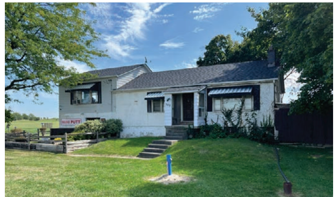
Mid 20th-century house-form building, constructed between 1954-1978 (ERA, 2025).
