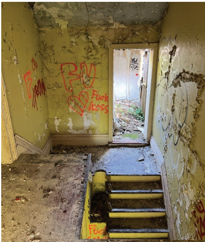
Looking towards the 20th-century rear addition from the second storey. Note the balustrade has been removed (ERA, 2025).
