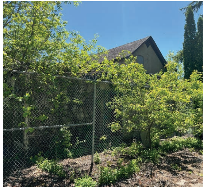
Looking towards the north elevation and one-storey addition at the rear of the 19th-century building (ERA, 2025).
