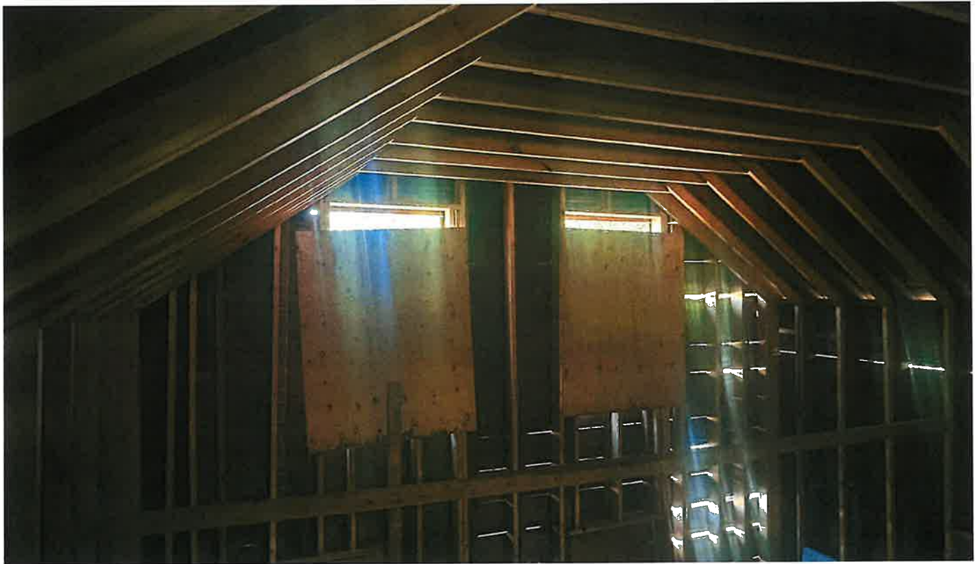
General view of upper floor of the house (looking West)
