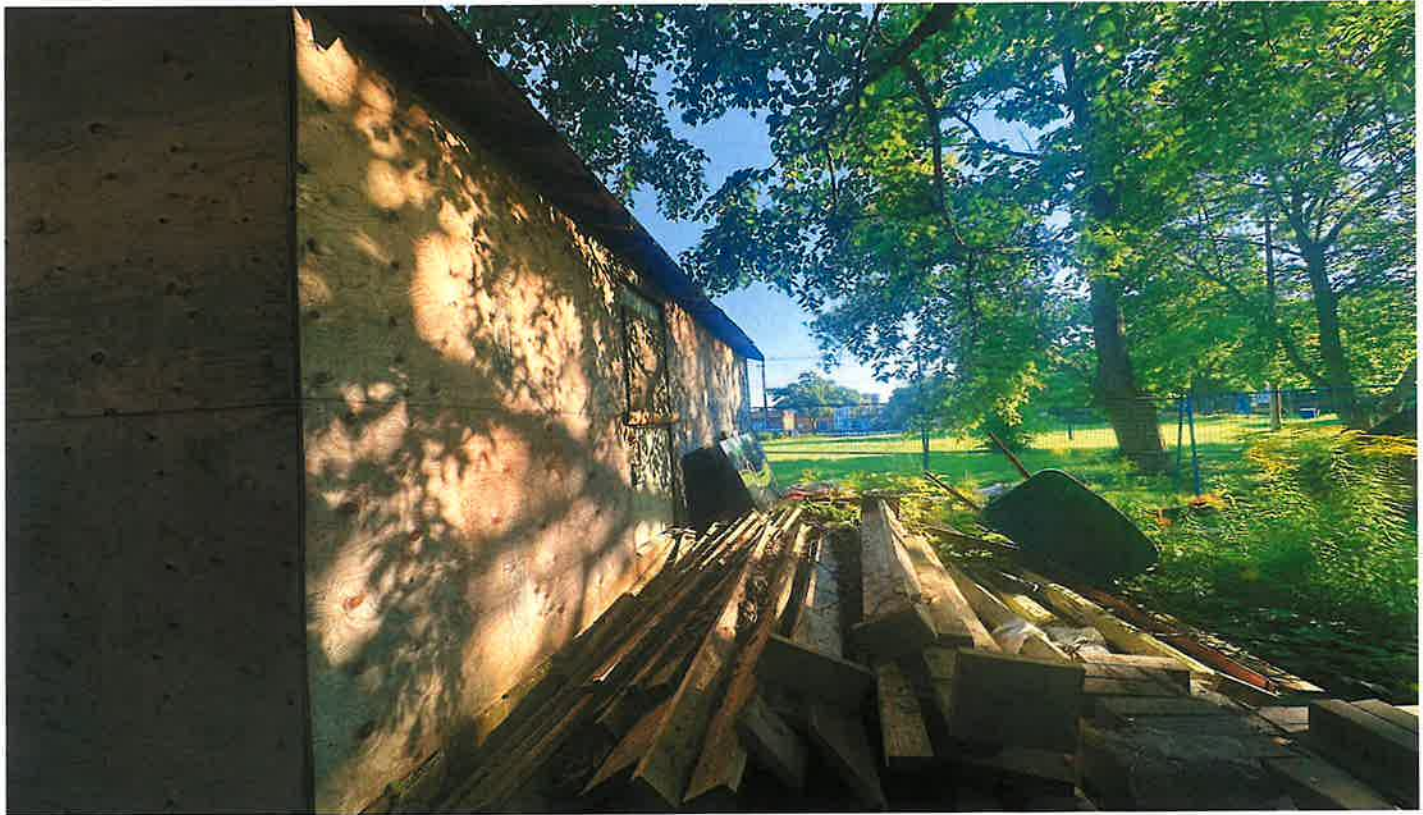
General view of south entrance to the house at the subject site (looking North)
