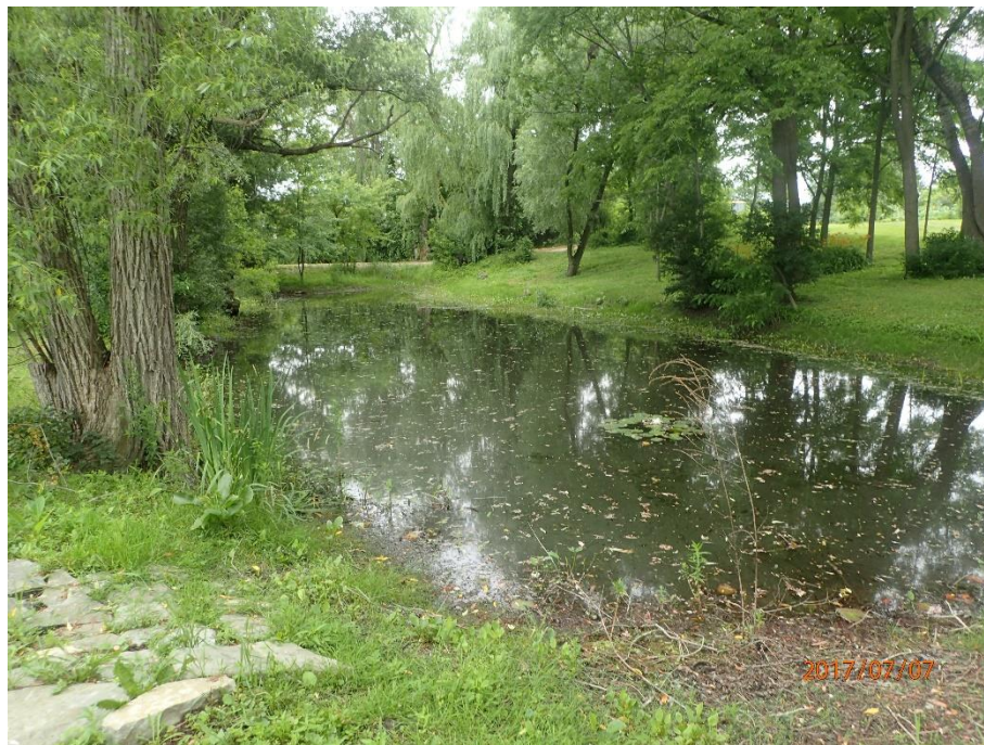
View of the earthen berm separating the offline pond located north of the channel.
