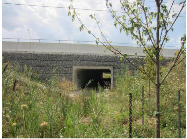
Photo <2>. Tributary 14W-W1-2 culvert under Bronte Road (Aug, 2012).
