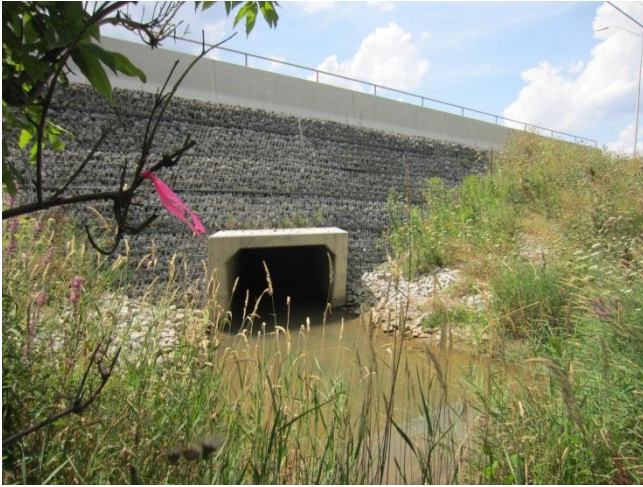
Photo <1>. Tributary 14W-W1-3 culvert under Bronte Road (Aug, 2012).
