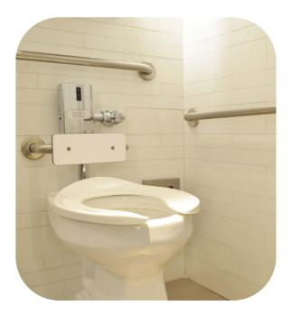
Measure the width of the clear transfer space from the edge of the water closet bowl or tank (whichever protrudes further) to adjacent obstruction.
