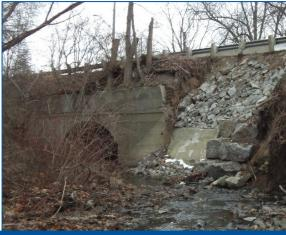
Collapse of the McCraney Creek Bridge's north-west wingwall in 2017 and subsequent emergency works to temporarily stabilize the slope
