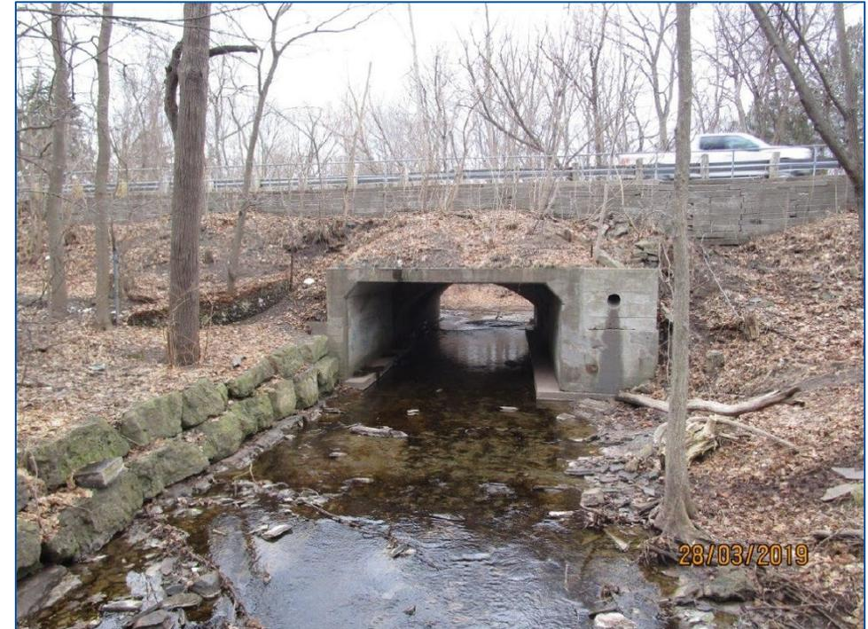
Box culvert extension of McCraney Creek Bridge along the downstream side (i.e., east side of Lakeshore Road West)
