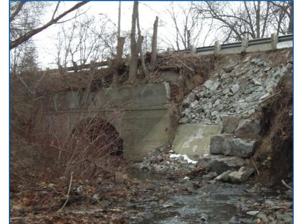
Collapse of the McCraney Creek Bridge's north-west wingwall in 2017 and subsequent emergency works to temporarily stabilize the slope
