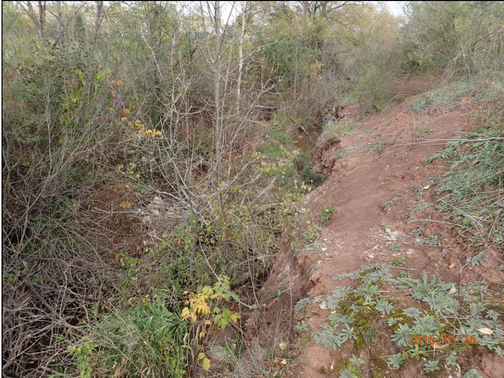
Photograph 11. October 26, 2016. Shrub and debris choked section of ditch, with high eroding banks. Approximately 1450 m west of 4th Line.
