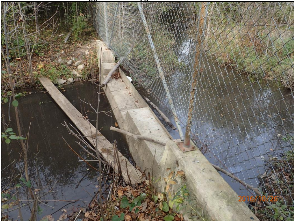
Photograph 8. October 26, 2016. Concrete weir in ditch. No apparent flow. Note dark water that suggests low oxygen.
