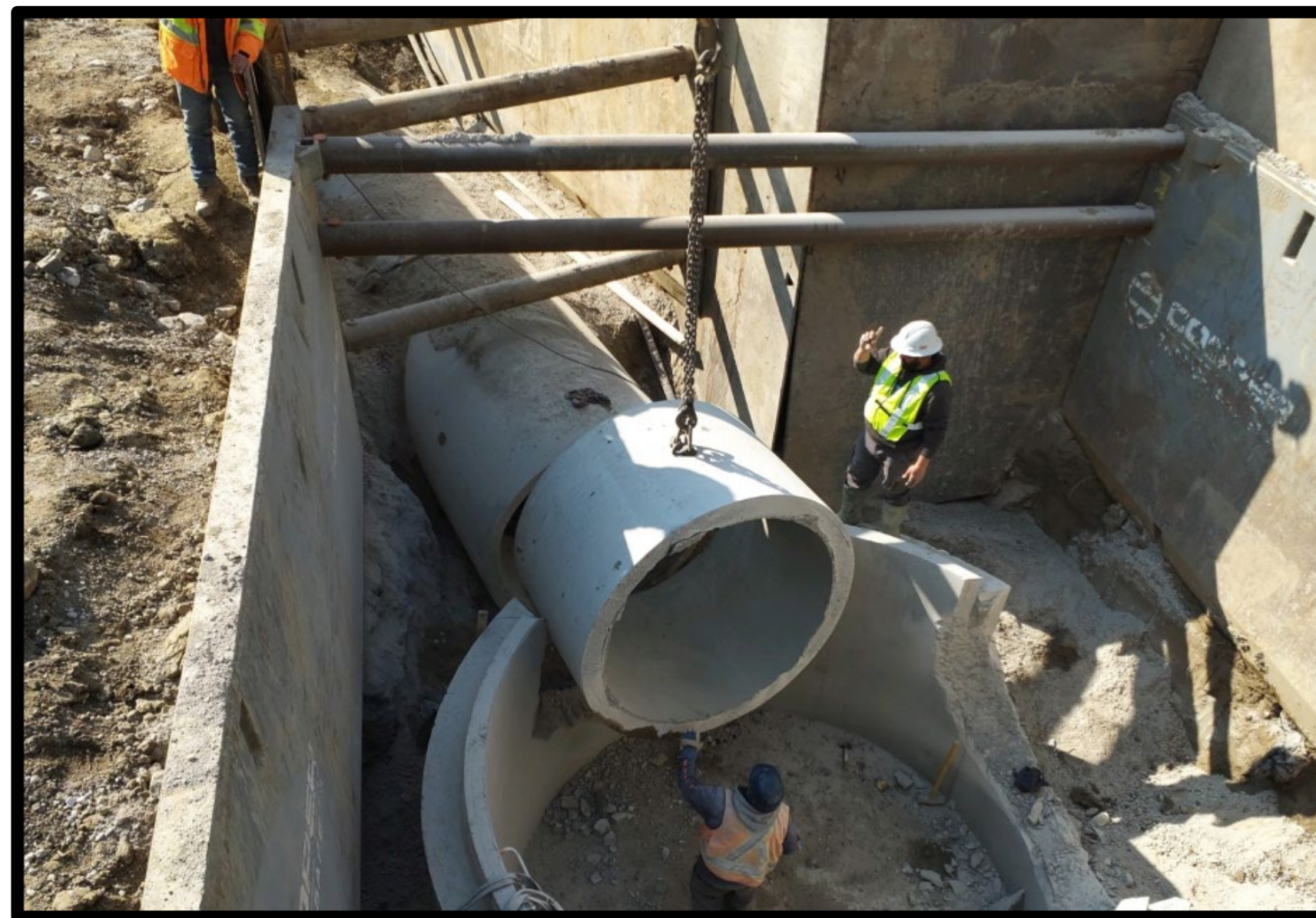
Alt 4A: Existing Storm Sewer Upgrades and Installation of New Storm Sewers
