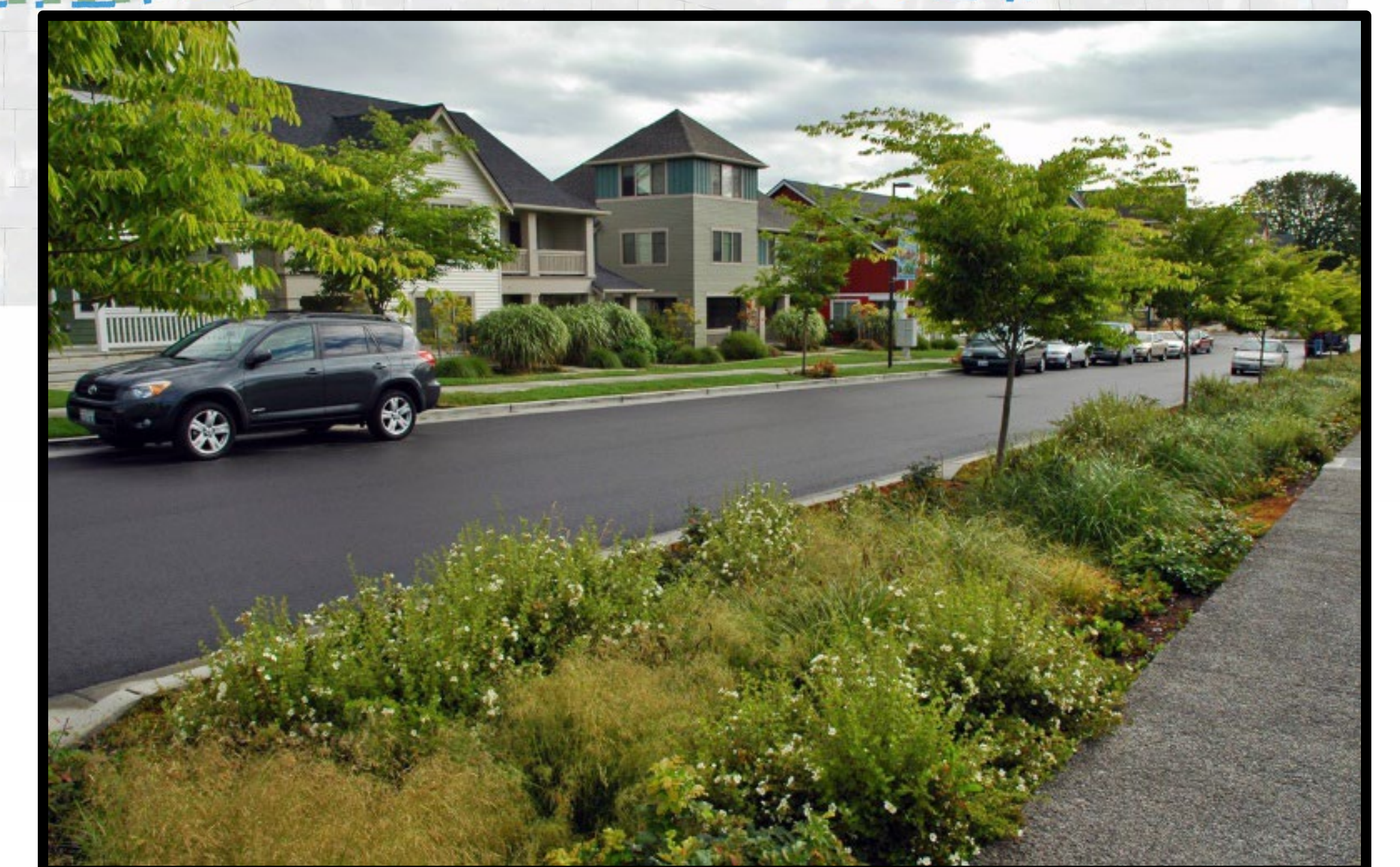
Alt 3B: Local (minor) Ditch System Improvements with LID/Green Infrastructure enhancement (Bioswale)
