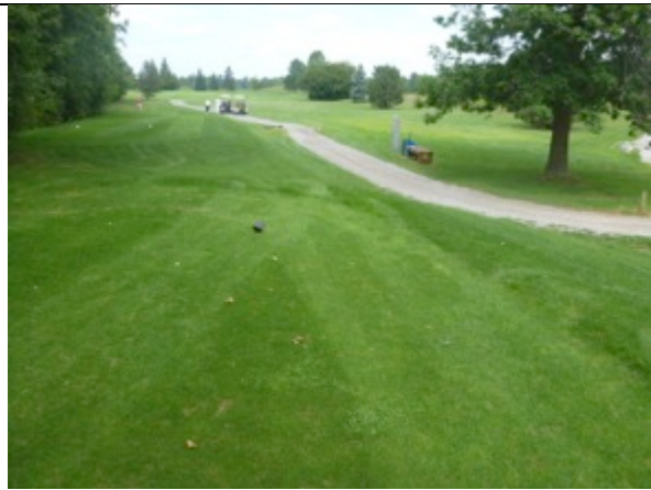
Plate 81 Gravel Cart Track
