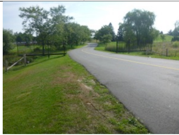
Plate 21 Asphalt Entrance off Bronte Rd
