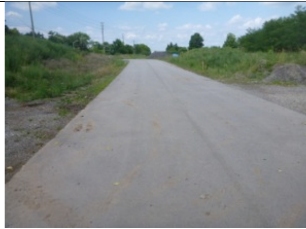
Plate 101 Asphalt Road to Maintenance Yard
