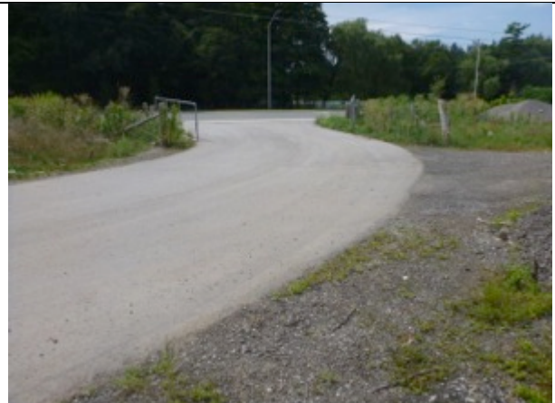
Plate 102 Maintenance Road Entrance
