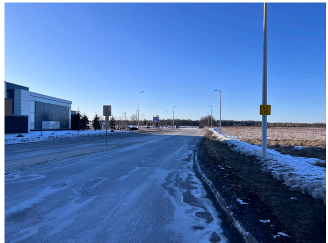
FIGURE 7. View of Glenorchy Road fronting ErinOakKids Centre for Treatment and Development
