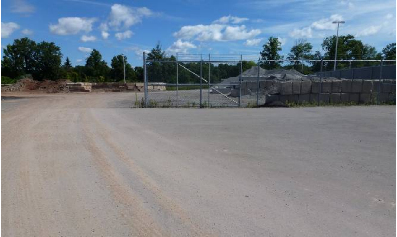
PHOTOGRAPH 1 HALTON REGION AGGREGATE YARD
