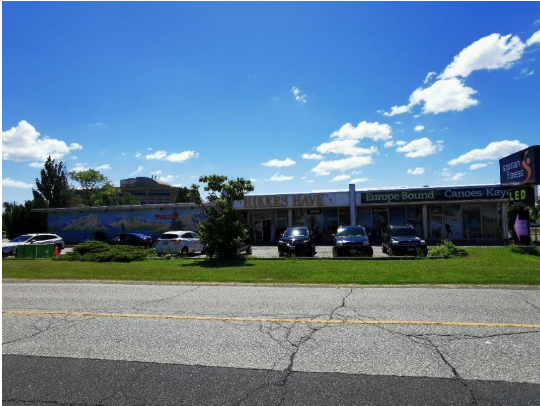
Photo 1: Frontage of the Site building, facing southeast.
