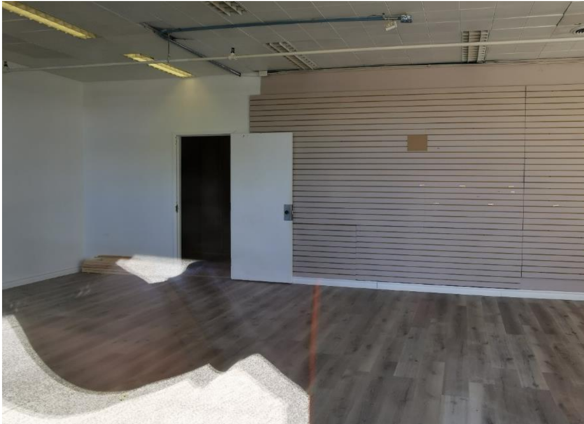
Photo 3: Interior of the Site building within Reno Max Lighting.
