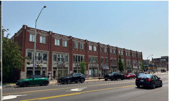
Left: Lakeshore Road West Right: Three storey main
