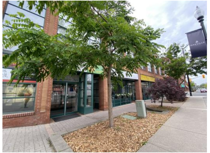
Photo 2: View of northwest side of the Site building from Church Street. Photograph taken facing south.
