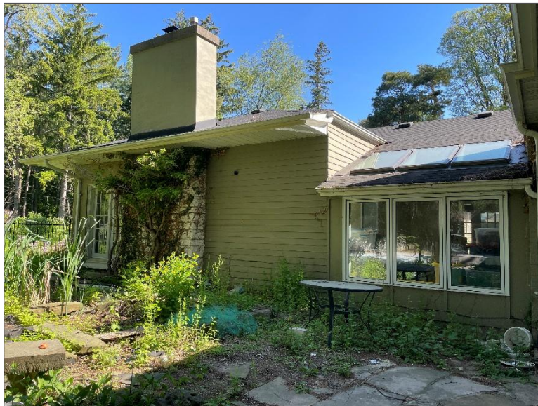
Photograph 4 – Site Building (southwest side).
