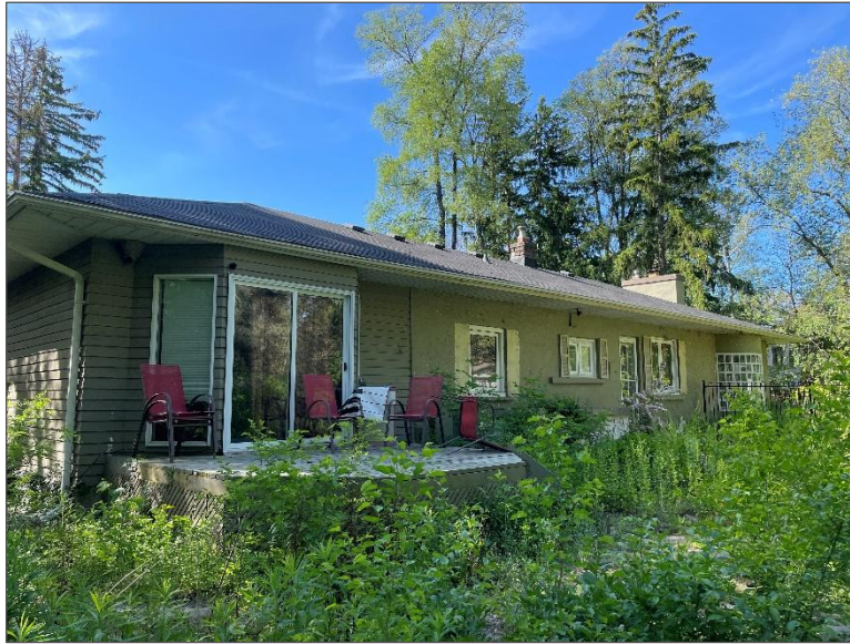
Photograph 3 – Site Building (northwest side).
