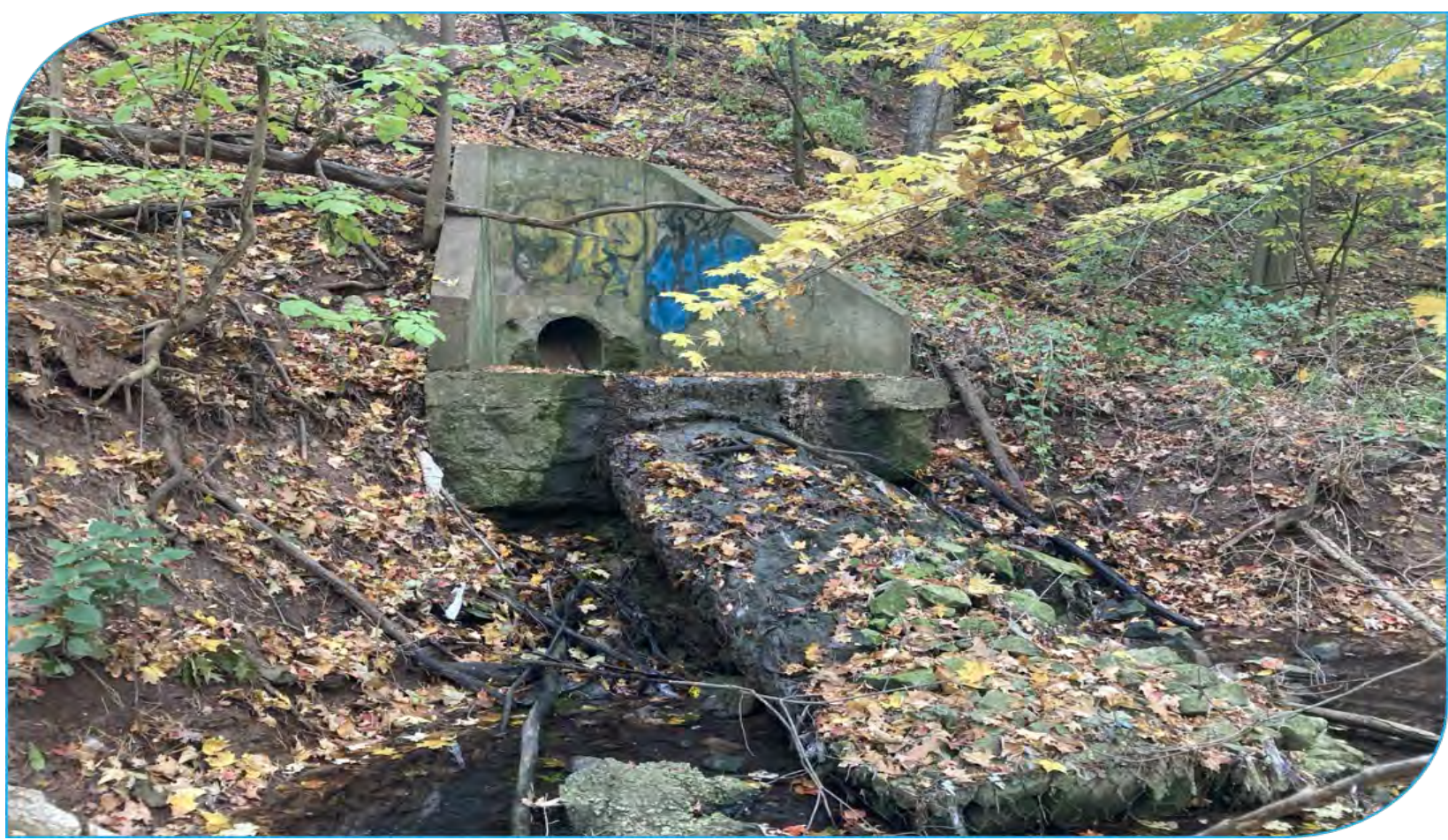
Site: E6 Score: 64 Issue: Perched outfall on valley slope, outfall drop structure suspended, scour pool below Risk: Private property; secondary infrastructure (outfall) Length: 50 – 100 m
