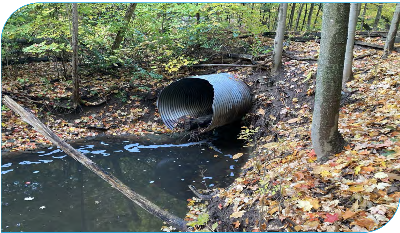
Site: E11 Score: 79 Issue: CSP culvert below trail, bottom corroded. Scour pool downstream. Buried sanitary sewer. Risk: Critical infrastructure (sanitary sewer), pedestrian path/crossing Length: 20 – 50 m
