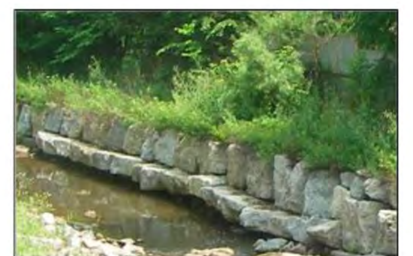
Armour Stone Wall with Brush Layer Concept
