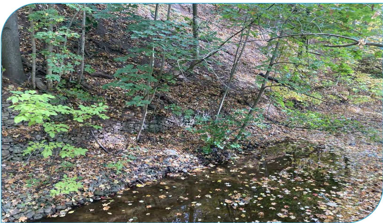
Site: E24 (new site) Score: 59 Issue: Valley contact/slope erosion. Gabion toe protection - fair condition (functioning, some wire failure at toe) Risk: Private property Length: 20 – 50 m
