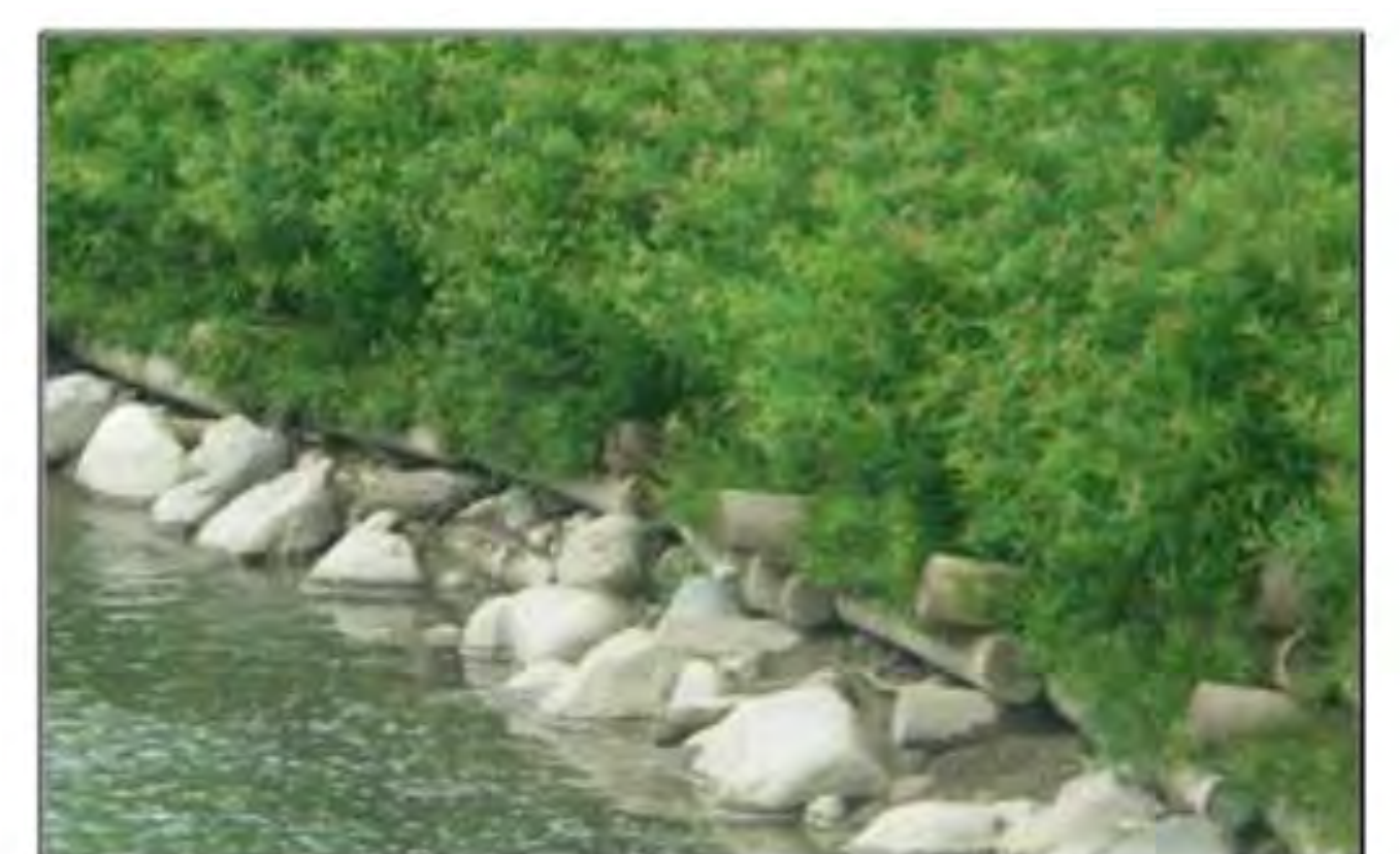
Live Log Crib Wall Concept
