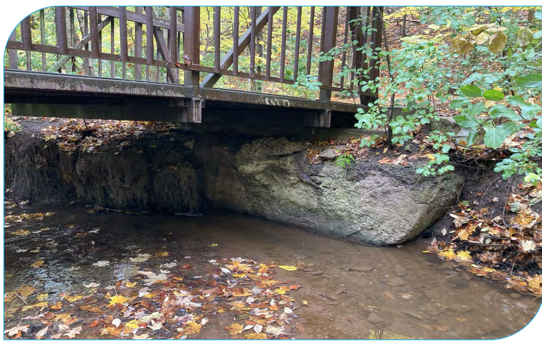
Site: E20 Score: 43 Issue: Erosion around pedestrian bridge crossing; footing exposed on the outer meander bend. Risk: Trail infrastructure including pedestrian trail and pedestrian bridge crossing Length: < 10 m
