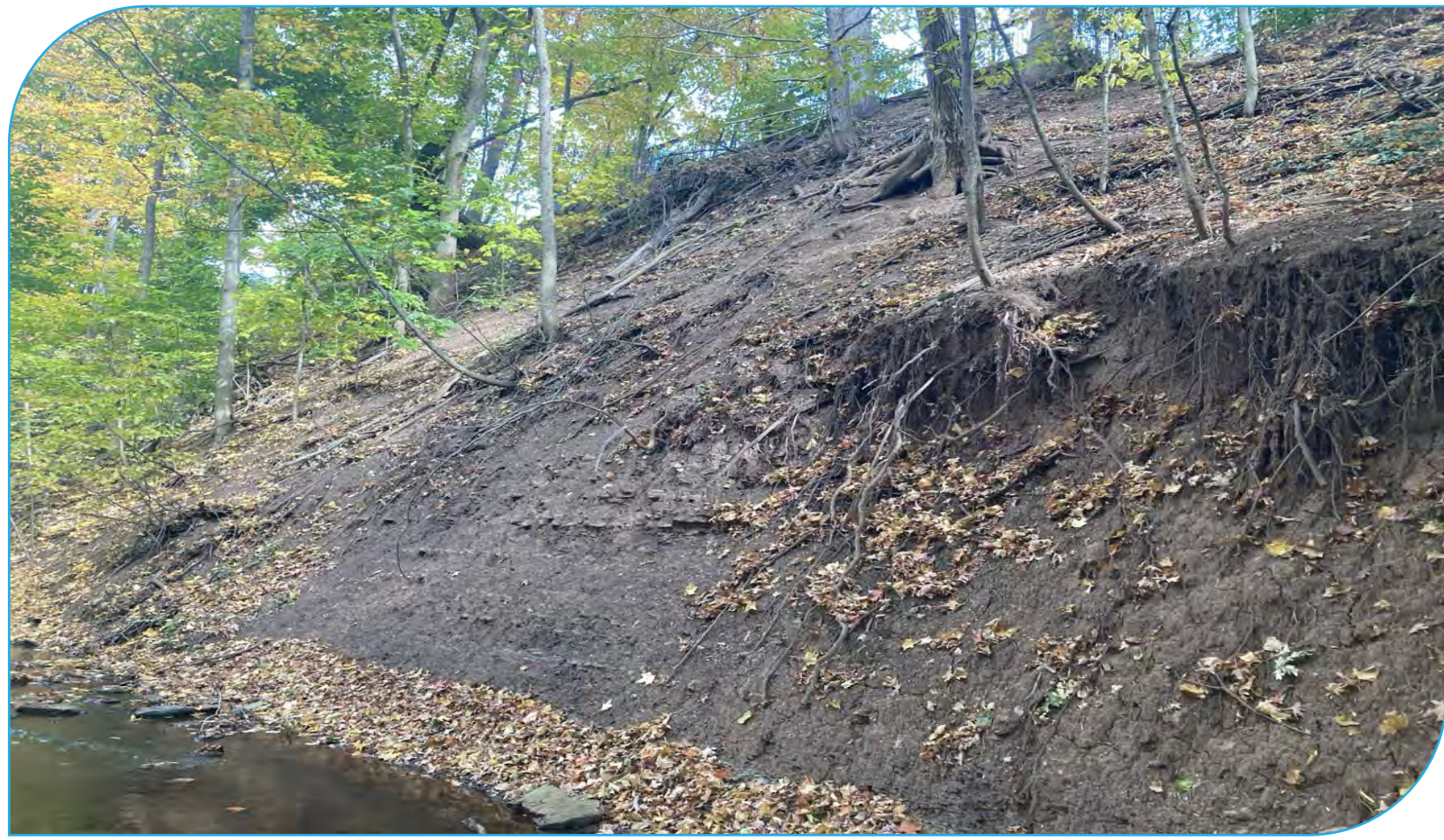
Site: E4 Score: 65 Issue: Valley wall contact and slope erosion. Gabion protection near upstream end of erosion is in poor condition (bottom tier corroded/emptied) Risk: Private property Length: > 100 m
