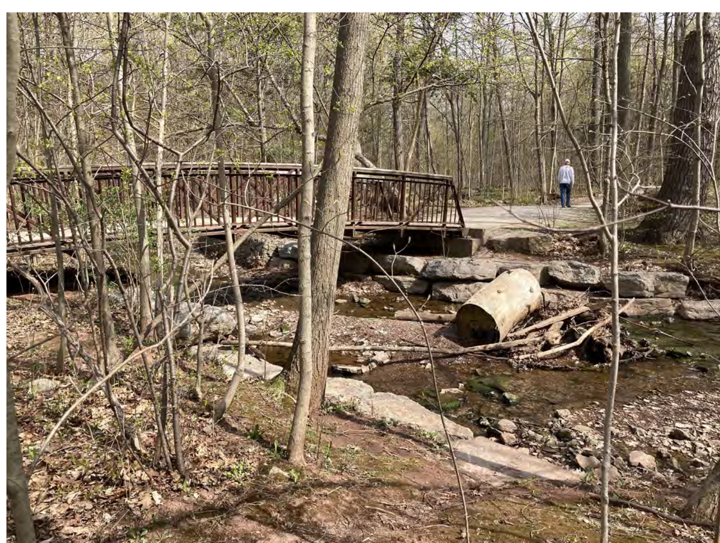
E5: Failing gabion baskets with downstream scour pool. Risk to pedestrian bridge/trail
