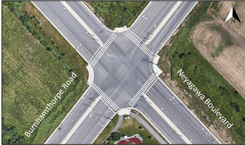
Figure 5: Intersection of Neyagawa Boulevard at Burnhamthorpe Road
