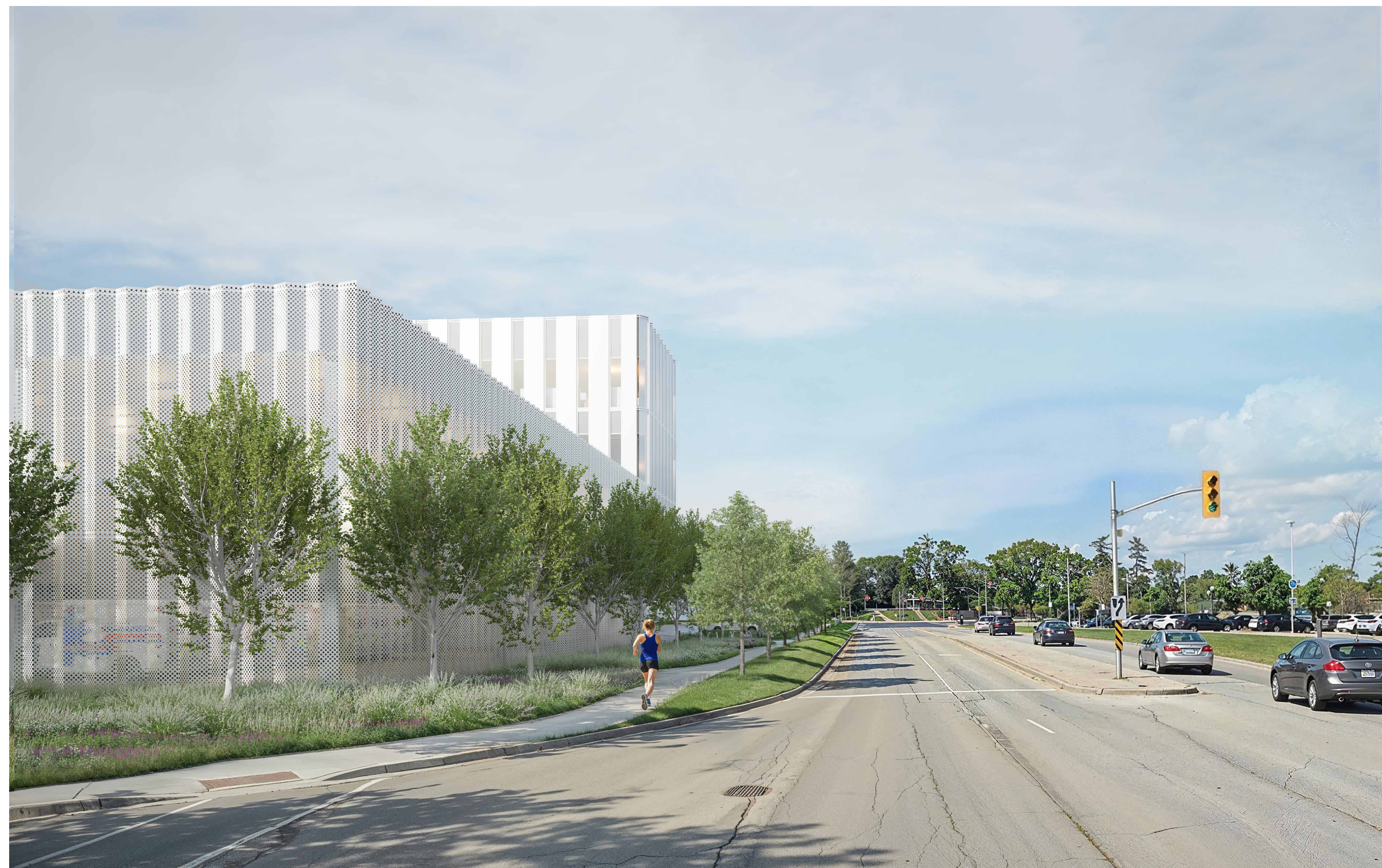
VIEW LOOKING WEST AT NORTH SERVICE ROAD NORTH SIDE.
