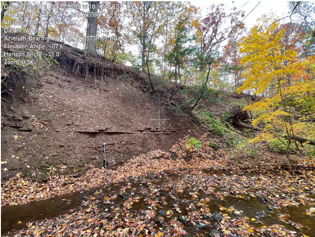
Photo 24. View of erosion in Zone A11-2 of the East Morrison Creek, looking Southwest. Trimble R10 in photo is 2-meters tall.
