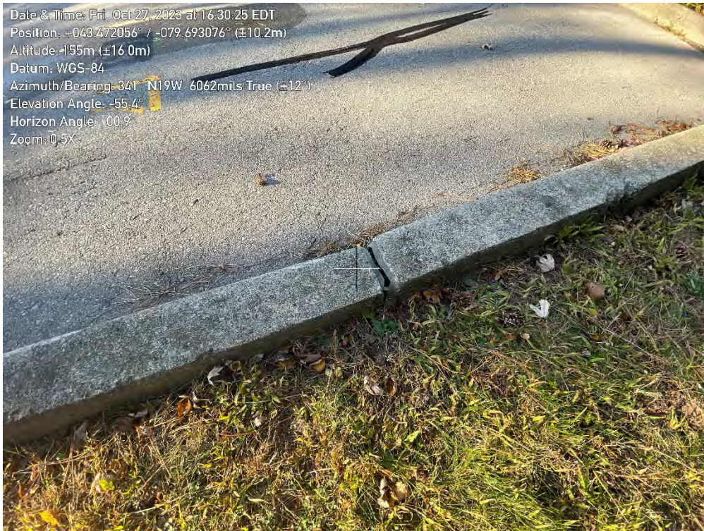
Photo 10. View of separating parking lot curbs at 1359 White Oaks Boulevard, slope crest of Zone A7, looking Northwest.
