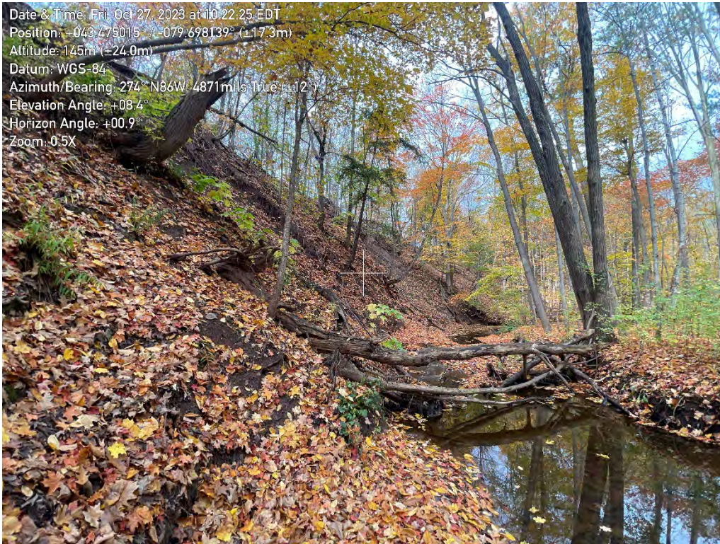
Photo 25. View of valley wall slope in Zone A13 of the East Morrison Creek, looking Northwest.
