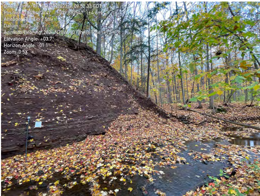
Photo 188. View of erosion in Zone A9 of the East Morrison Creek, looking Northwest. Trimble R10 in photo is 2-meters tall.
