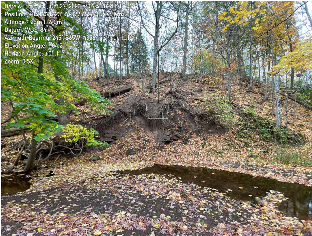
Photo 7. View of eroded slope in Zone A7 of the East Morrison Creek, looking Southwest.
