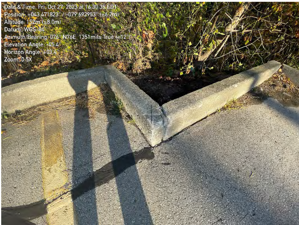
Photo 12. View of separating parking lot curbs at 1359 White Oaks Boulevard, slope crest of Zone A7, looking Northeast
