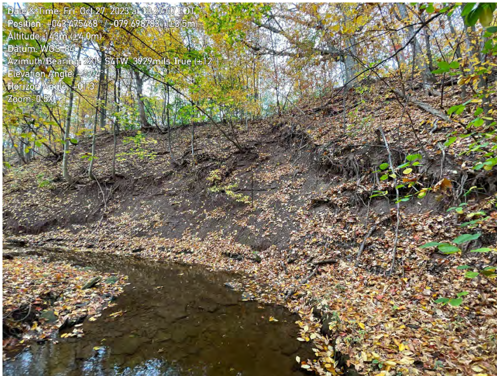
Photo 30. View of erosion in Zone A13 of the East Morrison Creek, looking Southwest.
