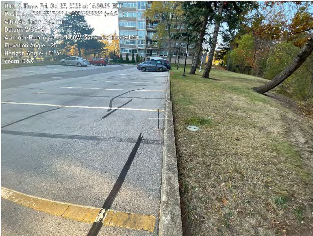
Photo 133. View of separating parking lot curbs at 1359 White Oaks Boulevard, slope crest of Zone A7, looking Northwest.
