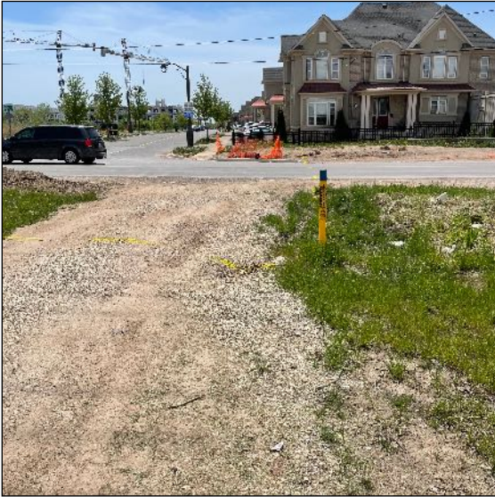
Image 1: Hazard area showing gas mains and disturbed roadway.
