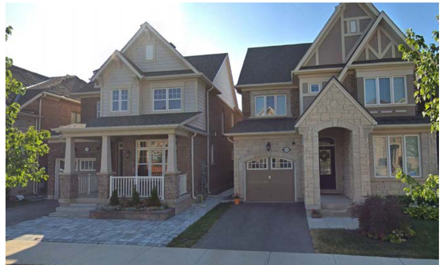
Fig. 6.4.2d - Image example of attached garages integrated into the main massing of the dwelling, behind the porch projection.
