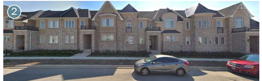
2 Existing townhouses on Carding Mill Trail, south of the NHS in Phase 4
