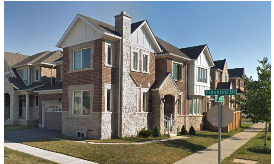
Fig. 6.5.1 - Image example of a corner lot dwelling in The Preserve that addresses both street frontages with the long elevation facing the flanking street.
