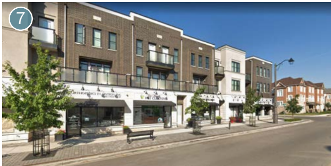
Live-work units on Preserve Drive, between Dundas St. W. and Betsy Drive.
