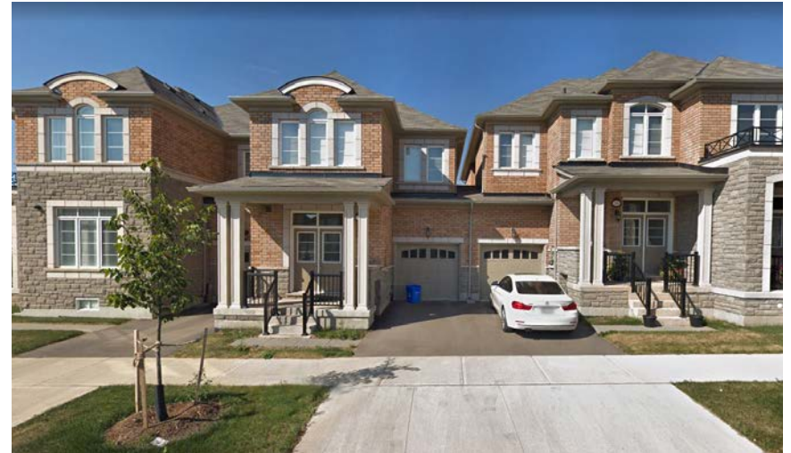
Fig. 6.3 - Existing street townhouses located on Carding Mill Trail, south of Phase 4.
