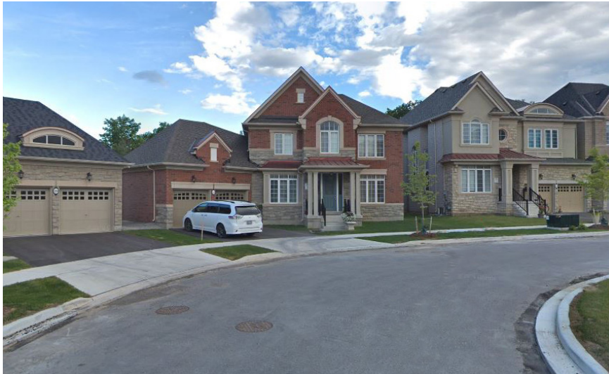
Fig. 6.5.2 - Image example of a view terminus dwelling in The Preserve, with a prominent architectural entry at the terminus view
