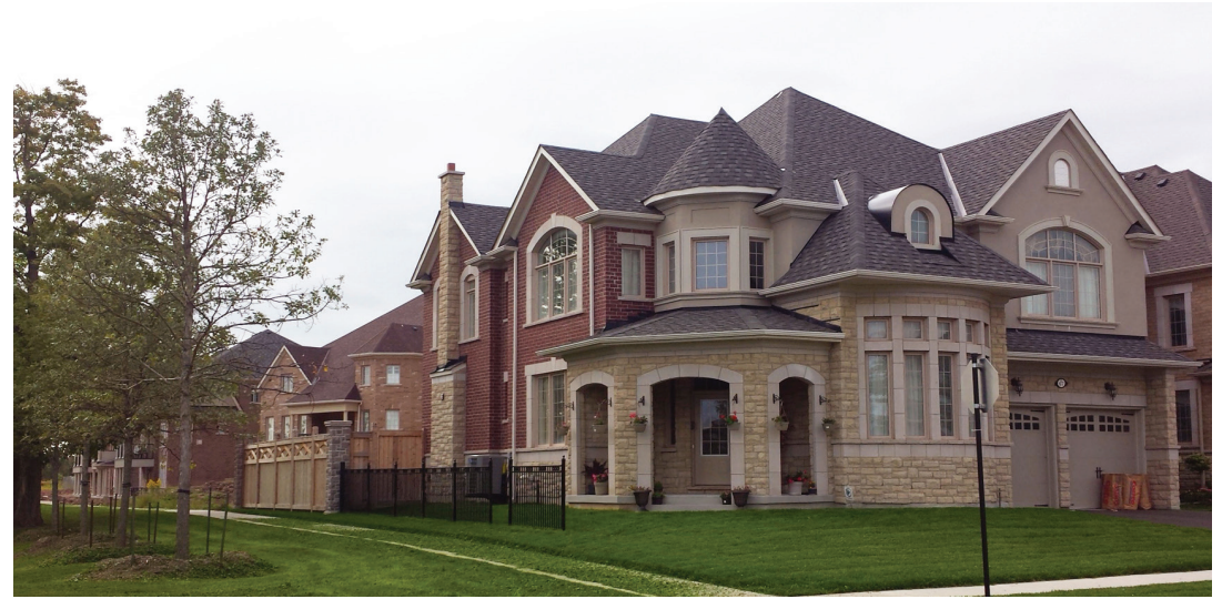
Fig. 7.8a - Example of a priority lot dwelling located at a corner that appropriately addresses both streets through architectural treatment (side-facing porch, wall articulation, windows, etc.)
