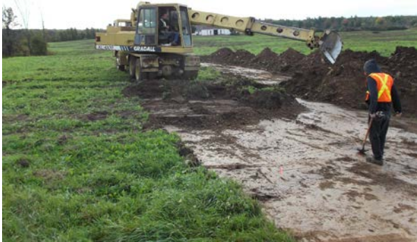
Plate 1. Gradall Stripping the Topsoil (view southwest)
