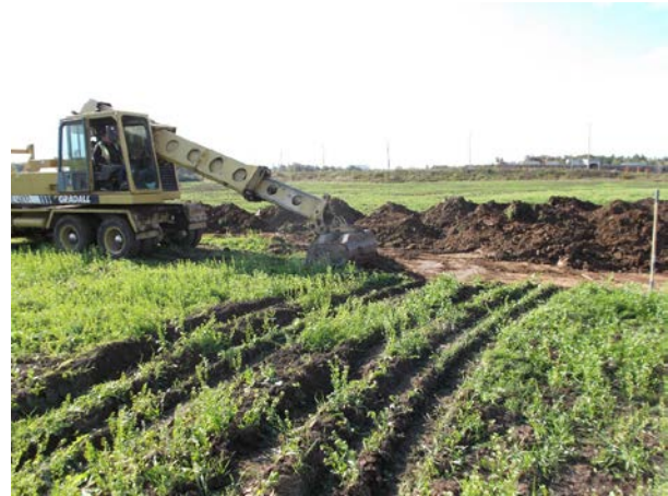
Plate 2. Gradall Stripping the Topsoil (view south)
