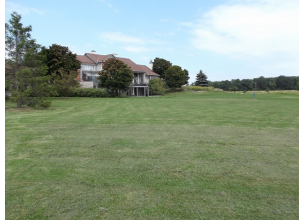
Plate 20. Southeast Residence, Landscaped Rear Lawn (view northeast)
