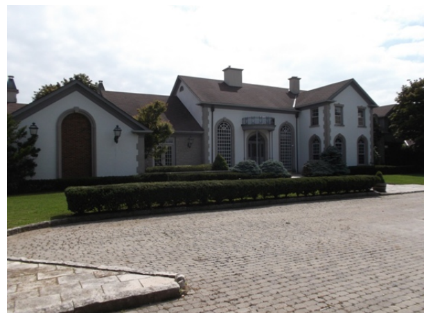
Plate 18. Southeast Residence, Front (view south)
