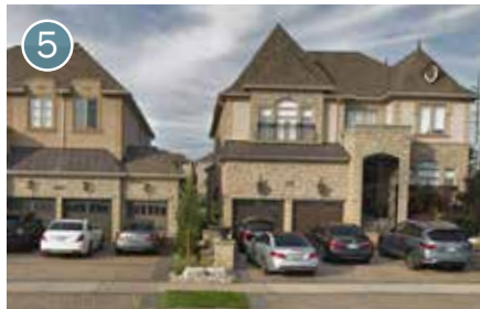
Fig. 2.2d - Single detached homes on Meadowridge Drive, south of the subject lands
