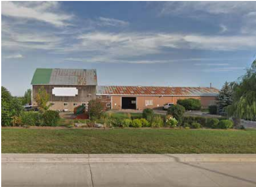
Fig. 6.6a - Existing view of the heritage-interest property facing north from Dundas Street (source: Google earth)
