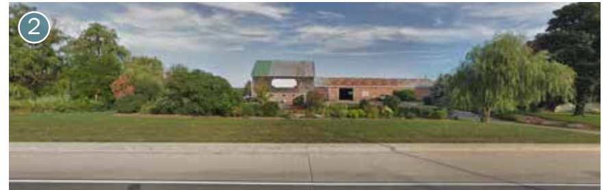
Fig. 2.2a - View facing north from Dundas St. E. toward the existing residential property and heritage farmhouse
