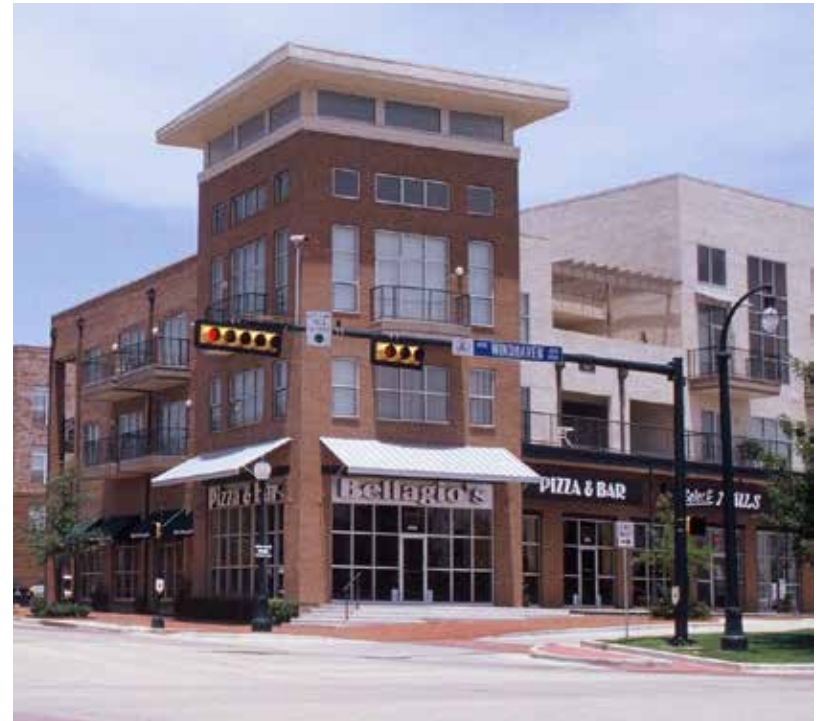
Fig. 6.2.2 - Image example of built form may comprise a mix of uses, including commercial, retail and residential. Prominent building massing and architectural treatment should be provided at the street edge.
