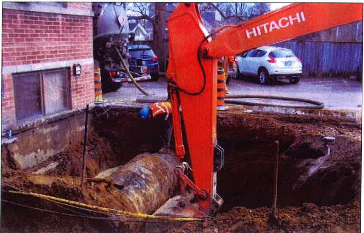
Photograph 2 Evacuation of Residual Fuel in Underground Storage Tank in Progress
