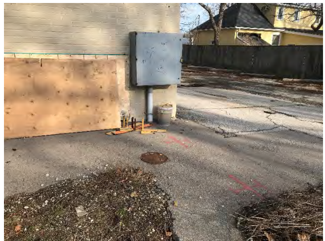
Photo 6: Existing recovery well located in the vicinity of the Former UST
