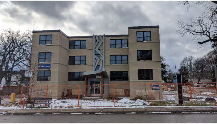
Photo 1: View from Front of Phase One Building
