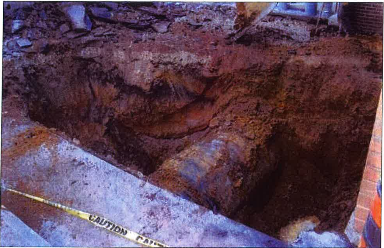
Photograph 1 View of Exposed Underground Storage Tank
