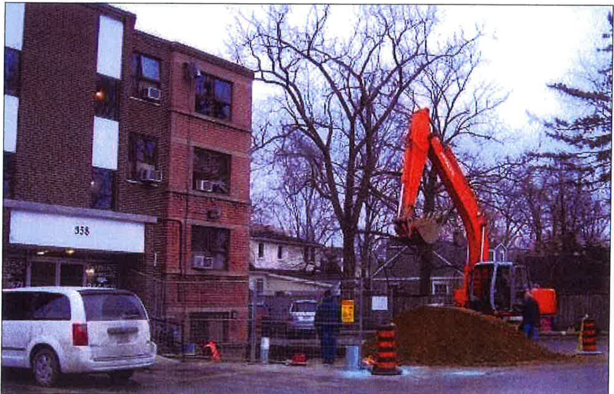
Photograph 6 Backfilling of Excavation Cavity in Progress
