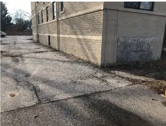
Photo 5: Existing well located near the Northeast corner of the Phase One Building
