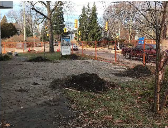
Photo 3: Four soil piles located in the Northern Portion of the Phase One Property
