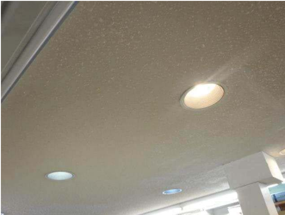
Water damage repair
