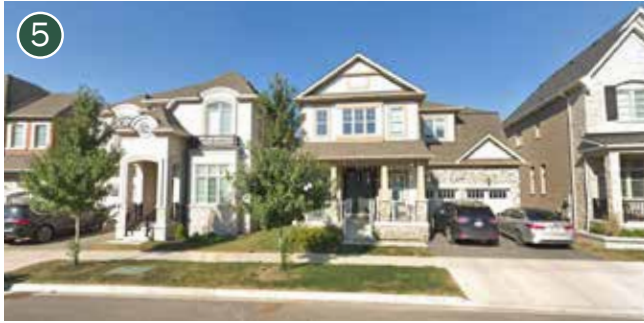
Existing single detached houses on Preserve Drive, south west of the Star Oak Development subject lands.
