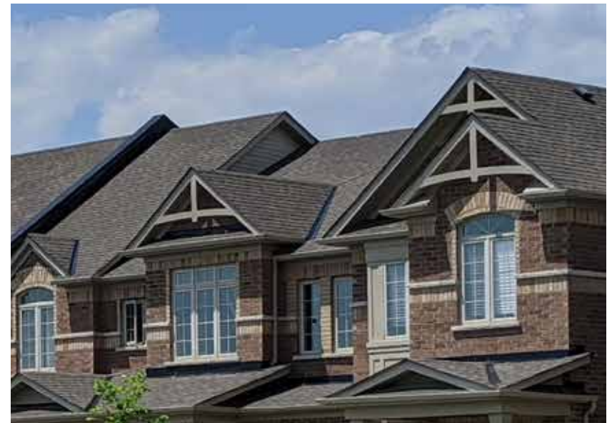
Traditional roof design
