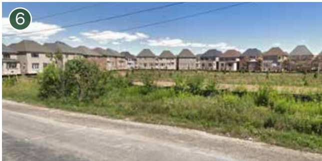
Existing single detached houses under construction backing onto NHS channel along east side of Sixth Line, south east of the Star Oak Development subject lands.
