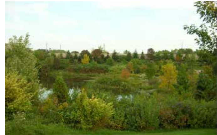
Fig 6.1.1c - Example of a SWM pond that functions as an important ecological and community amenity through a naturalized planting strategy and controlled pedestrian interaction.
