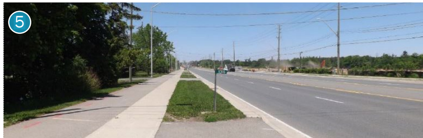
View facing north on the west side of Bronte Road
