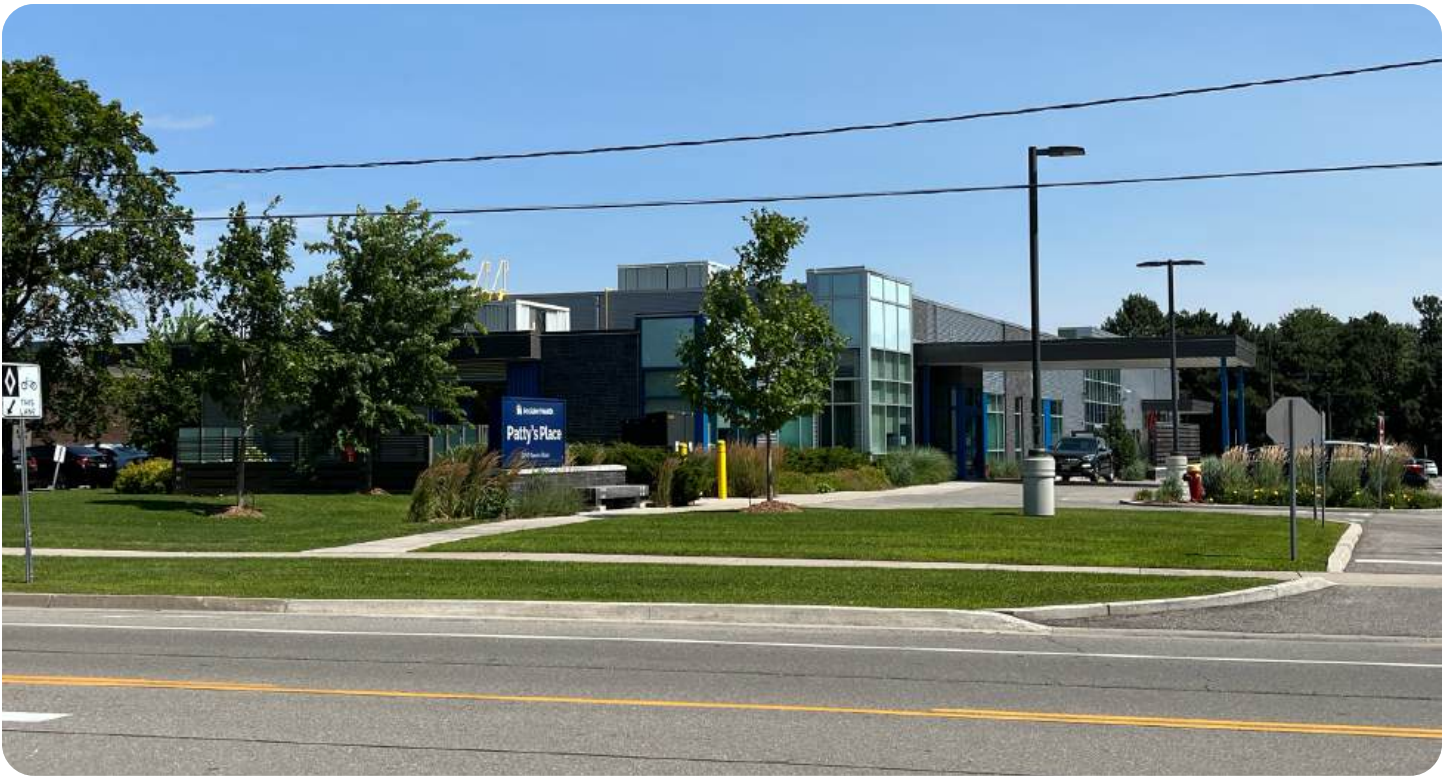
Subject Site, View looking south from Speers Road
