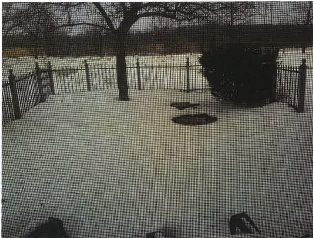
View of septic tanks, east of Residence B
