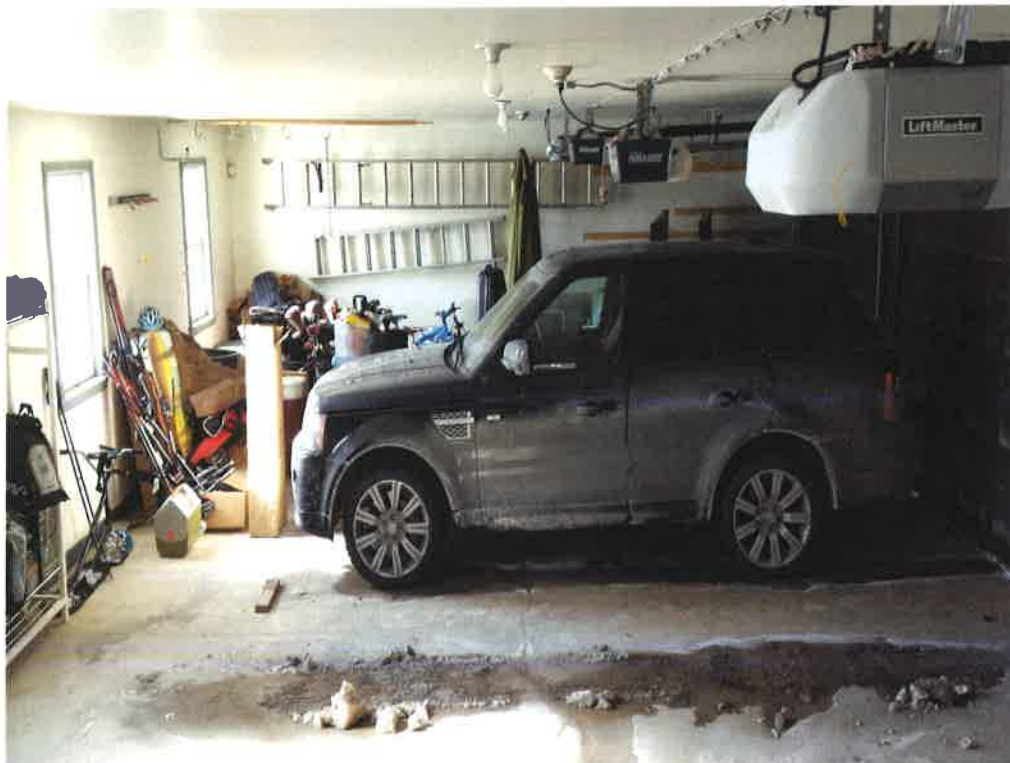
General view of garage in Residence A
