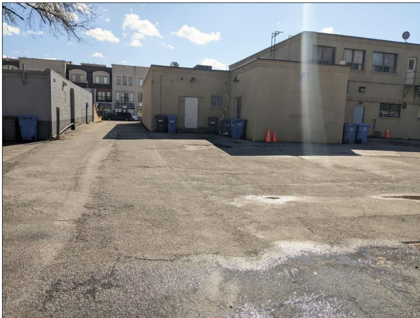
Image 4: View of the east half of the property and rear of the existing building fronting Lakeshore Road West, looking southeast.
