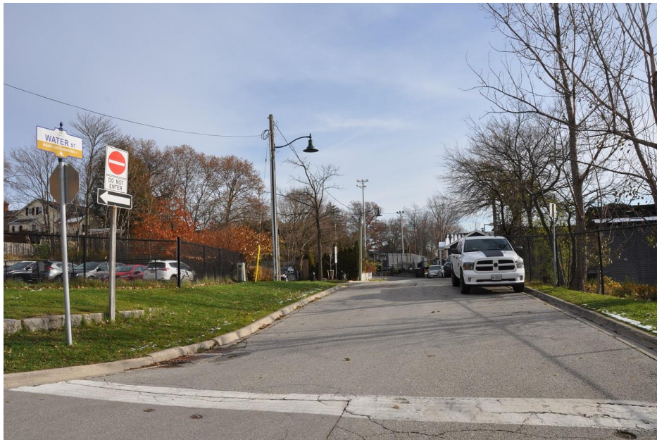
4.1.4.D. – Access along Water St.
