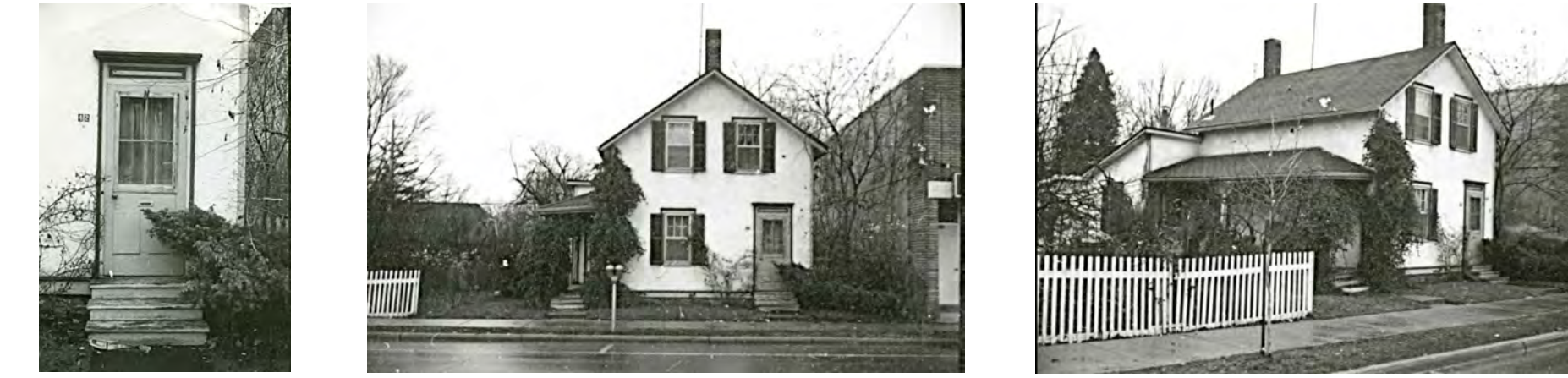
EXISTING HERITAGE HOUSE
