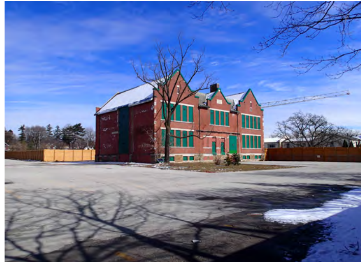
Figure 22: Northwest view of Oakville Trafalgar High School and context, 2018 (EVOQ)
