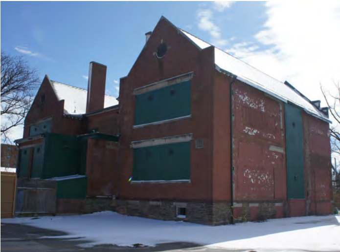
Figure 7: East (rear) elevation of Oakville Trafalgar High School, 2018 (EVOQ)
