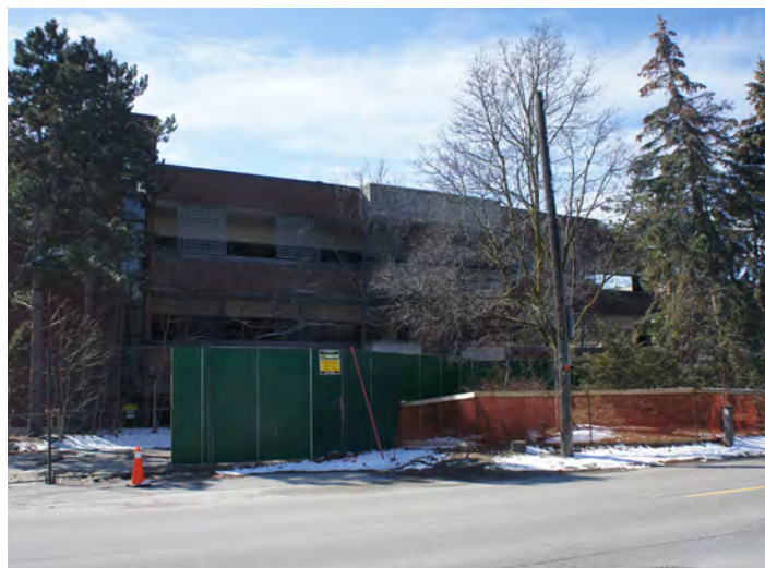
Figure 19: Facing westwards along Allan Street, rear of Parking Structure, 2018 (EVOQ)
