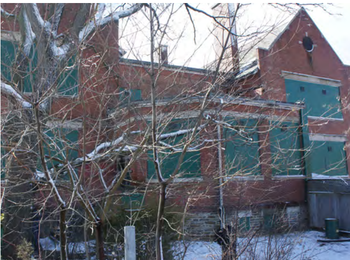
Figure 9: East (rear) elevation of Oakville Trafalgar High School, 2018 (EVOQ)
