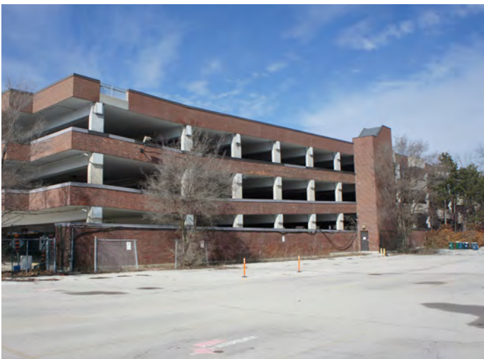
Figure 25: Facing northwards within Subject Property, towards Parking Structure, 2018 (EVOQ)
