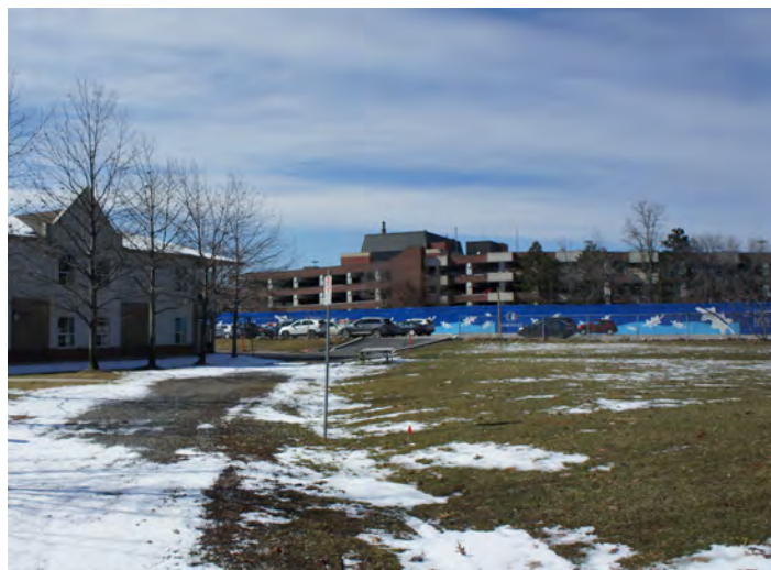
Figure 18: Looking northwards from Allan Open Space with Wyndham Manor Long Care Centre (left) and Parking Structure (center), 2018 (EVOQ)
