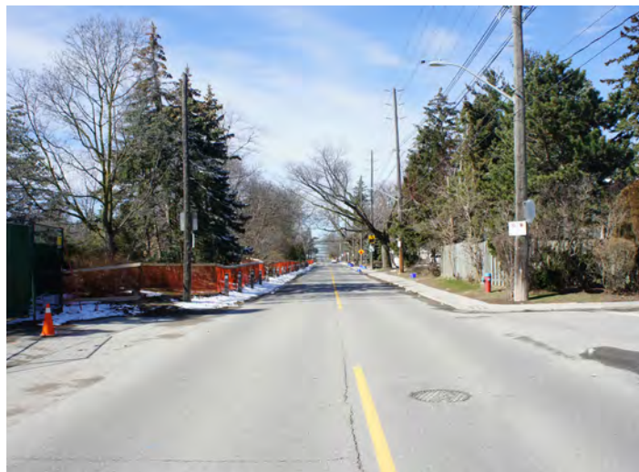
Figure 20: Looking northwards along Allan Street, Subject Property (left), 2018 (EVOQ)
