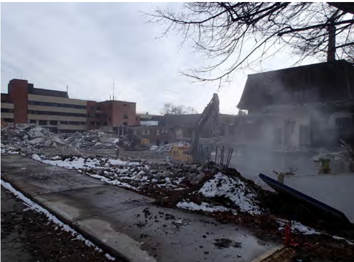
Figure 30: Looking southwards to Subject Property from MacDonald Street, 2018 (EVOQ)
