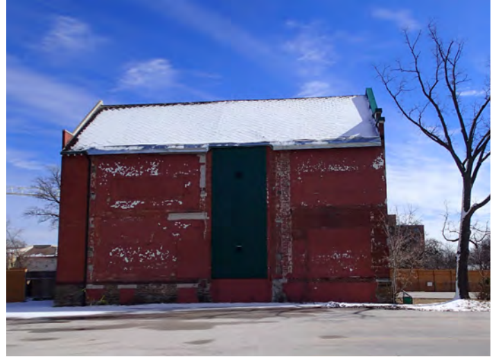
Figure 6: North (side) elevation of Oakville Trafalgar High School, 2018 (EVOQ)
