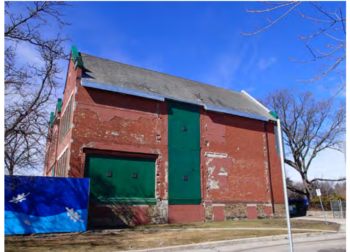
Figure 8: South (side) elevation of Oakville Trafalgar High School, 2018 (EVOQ)
