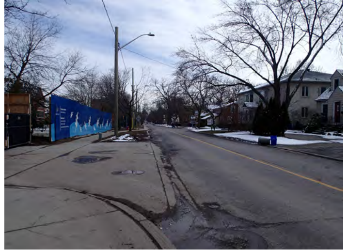
Figure 29: 289 Looking southwards along Allan Street, Subject Property on the left, 2018 (EVOQ)
