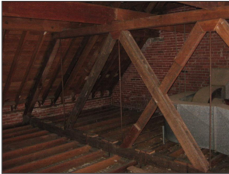
Photograph 6: Heavy timber truss (2016 Assessment)
