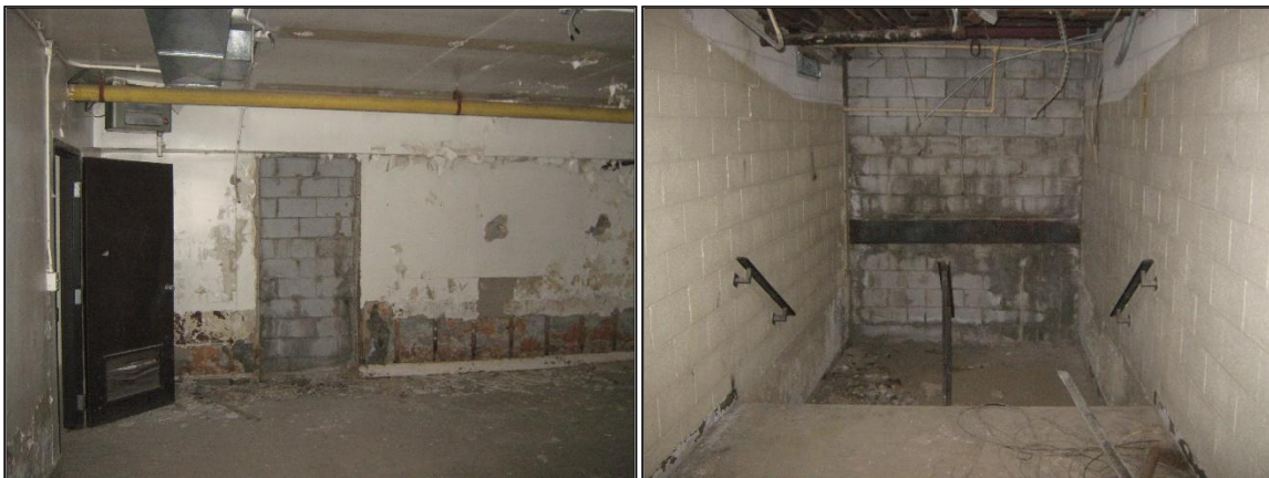
Photograph 3: Infilled concrete block wall (2016 Assessment)
