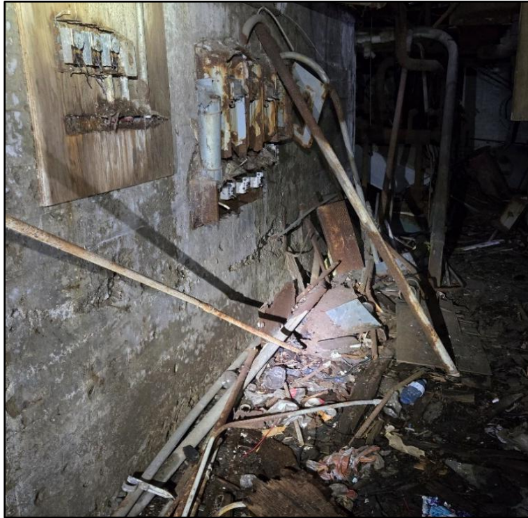
Photograph 5: Condition of basement foundation wall (August 2025 assessment)
