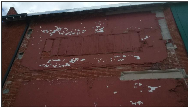
Photograph 14: Exterior beam pockets in load bearing wall (2016 Assessment)
