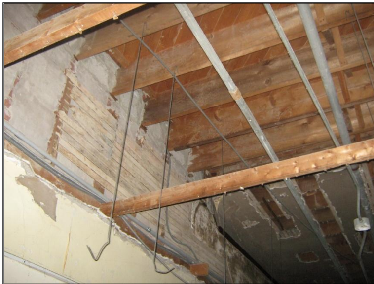
Photograph 9: Floor framing (2016 Assessment)
