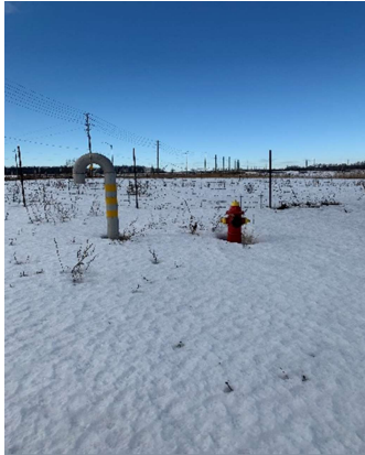
Picture 3: View of the Phase One Property, facing west.
