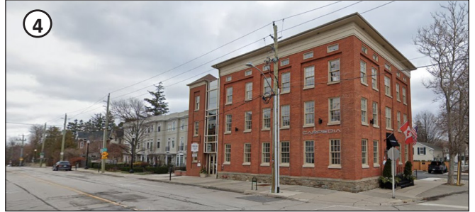
4 Commercial property to the east
