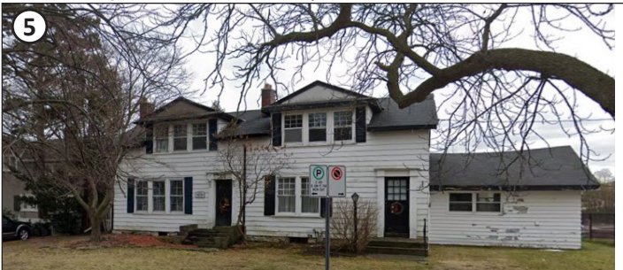
5 Semi-detached properties to the south
