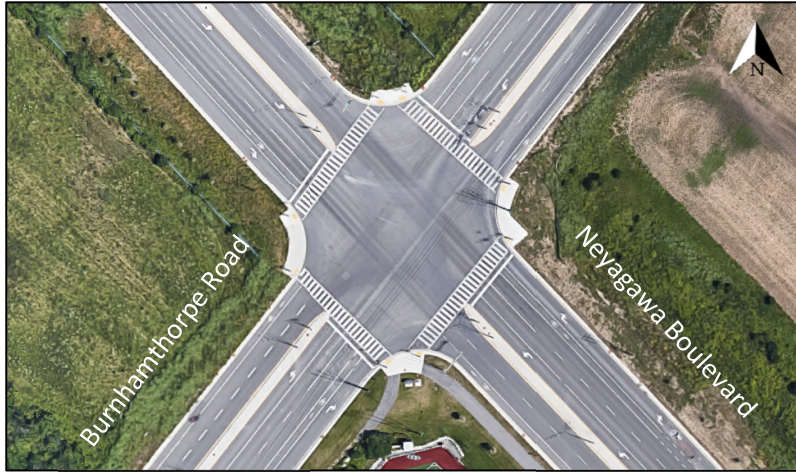
Figure 3: Intersection of Neyagawa Boulevard at Burnhamthorpe Road
