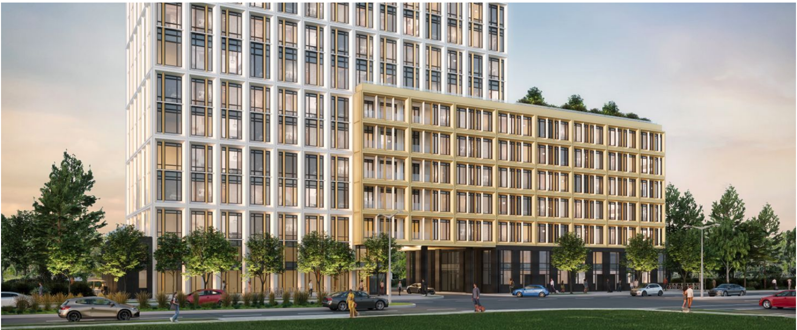
Proposed public realm interface along Sixth Line (Dundas Street to the right)
