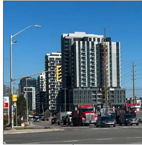
3065-3315 Trafalgar Rd & 345 Wheat Boom Dr - constructed 14, 16, 20, 20 storeys
