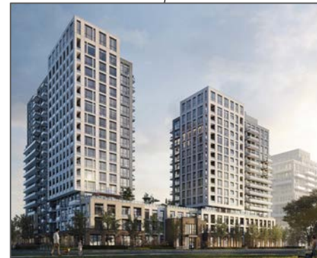
377-411 Dundas St E - under construction 15, 16, 17 storeys
