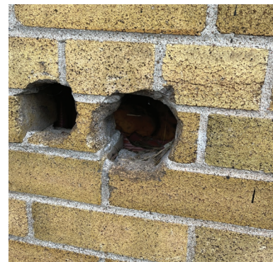
A section at the base of the brick wall on the south elevation showing signs of destructive testing (ERA, 2024).
