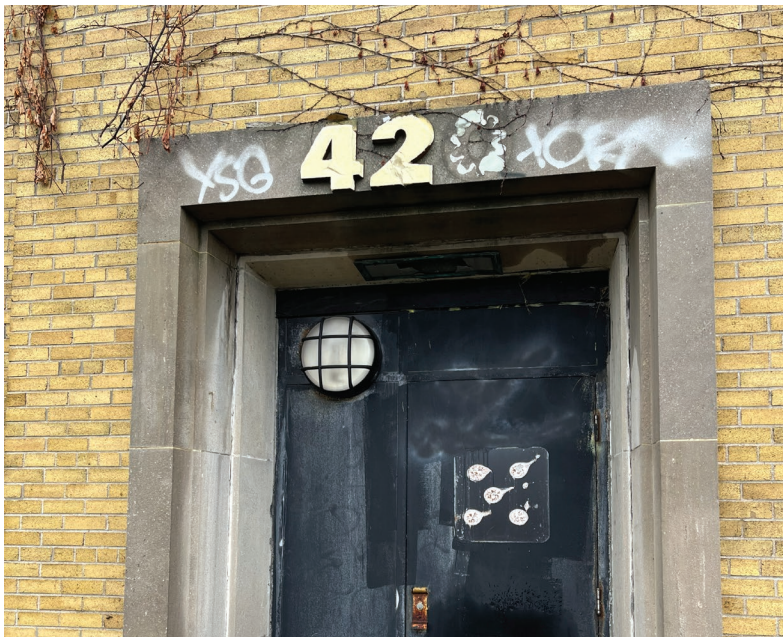
Stone portico main entrance is in fair condition with areas of poor condition showing delamination, mortar loss, staining, and graffiti (ERA, 2024).
