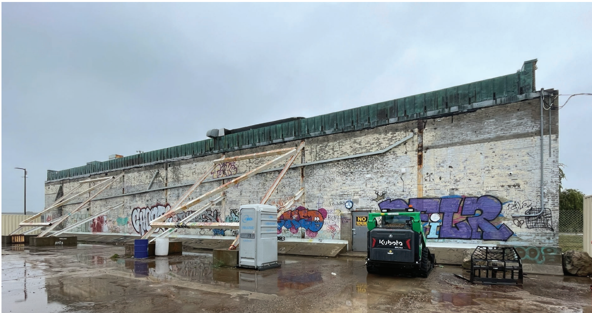
Looking north toward the southern elevation of the building. Following the demolition of the factory buildings in 2011, steel shoring was installed to support what was originally an interior wall (ERA, September 23, 2024).
