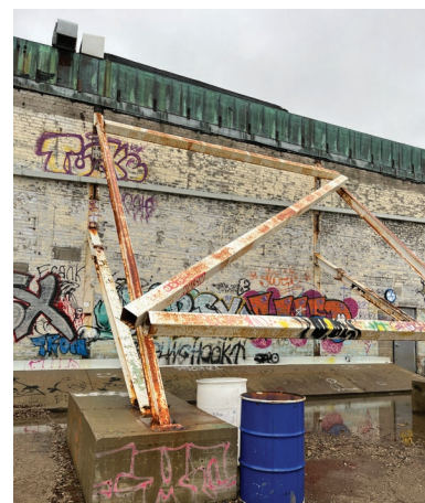
Bricks on south elevation and temporary steel shoring is in poor condition (ERA, 2024).
