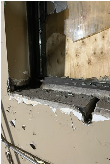
Missing drywall showing concrete block underneath; windows in defective condition showing broken glazing (ERA, 2024).
