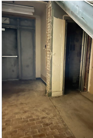
Metal door at the main entrance is in poor condition; missing drywall showing brick underneath (ERA, 2024).
