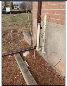
Photograph 2: Vent and Filler Pipe at northwest exterior wall of residential structure
