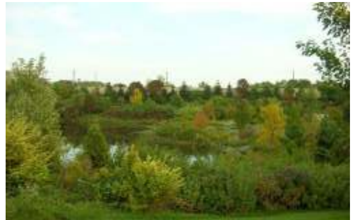
Fig 6.1.1b - Example of a SWM pond that functions as an important ecological and community amenity through a naturalized planting strategy and controlled pedestrian interaction.
