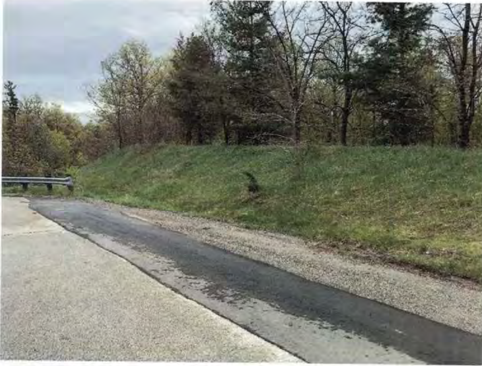
West Slope – Looking south, Cross Section C
