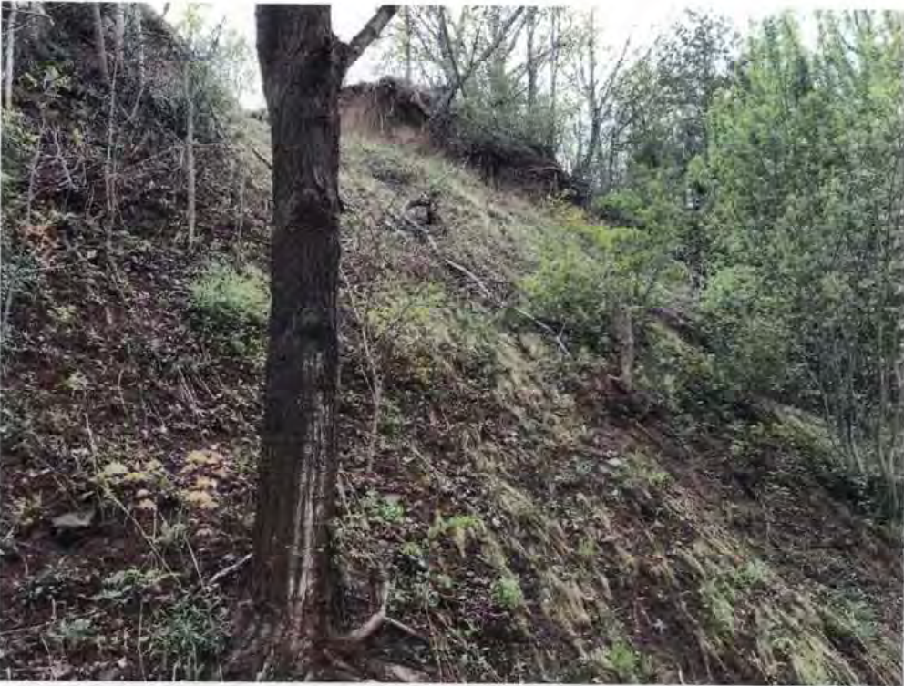
Sixteen Mile Creek Slope – Looking Northwest, Cross Section C
