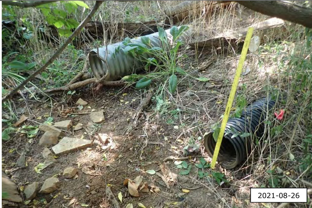
Upstream view towards the upstream extent of the ravine feature. The two culverts, left to right, were approximately 0.40 m and 0.30 m in diameter.
