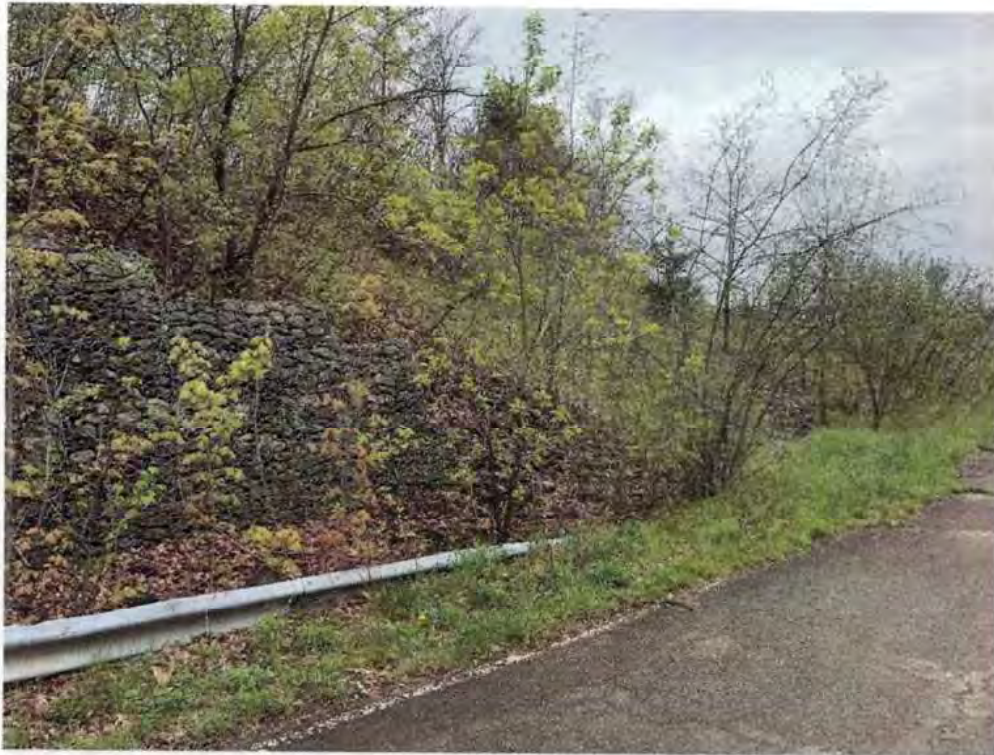
West Slope – Looking North, Gabion Retaining Wall
