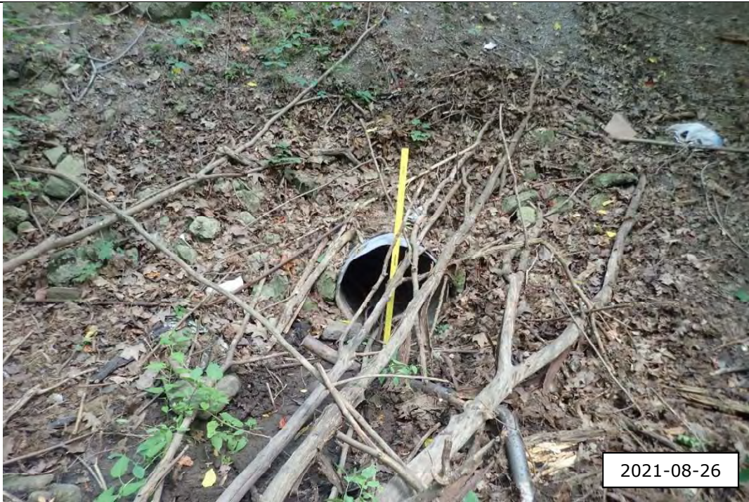
Photo taken at the downstream extent of reach, facing downstream. The culvert connected to Reach GC2 and was approximately 0.5 m in diameter.
