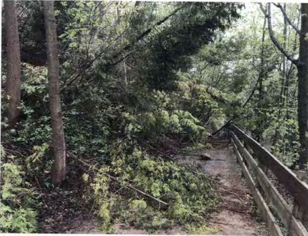
Sixteen Mile Creek Slope – Looking Southwest, slope overburden erosion impeding path, Cross Section B
