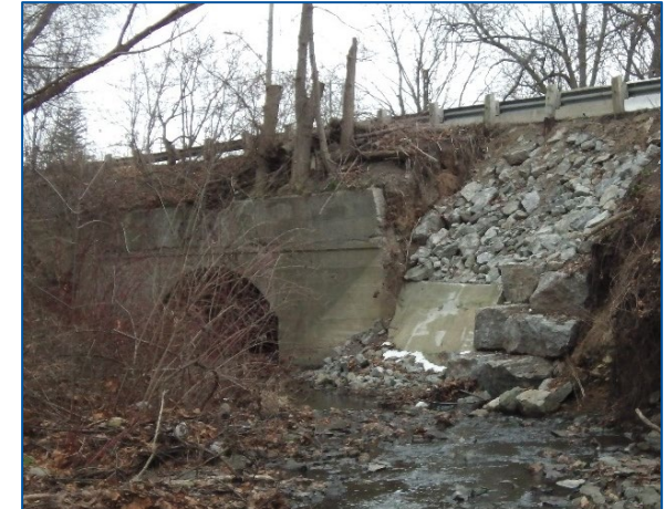
Collapse of the McCraney Creek Bridge's north-west wingwall in 2017 and subsequent emergency works to temporarily stabilize the slope
