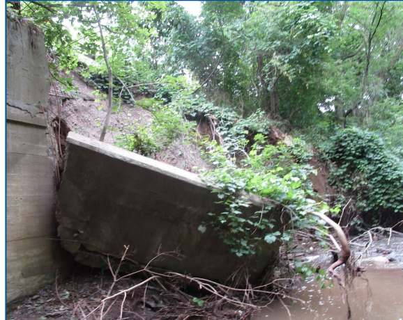
Collapse of the McCraney Creek Bridge's north-west wingwall in 2017 and subsequent emergency works to temporarily stabilize the slope
