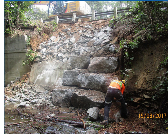
Collapse of the McCraney Creek Bridge's north-west wingwall in 2017 and subsequent emergency works to temporarily stabilize the slope
