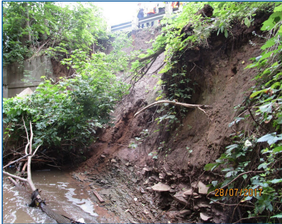
Collapse of the McCraney Creek Bridge's north-west wingwall in 2017 and subsequent emergency works to temporarily stabilize the slope
