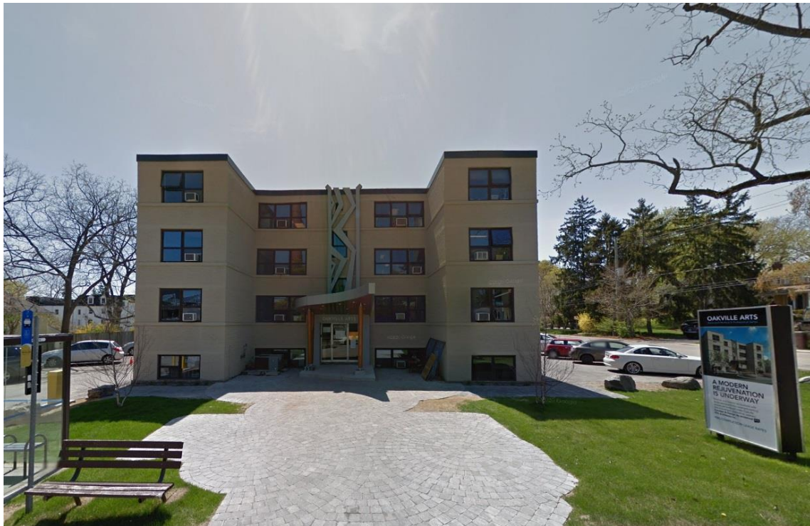
4.1.5.1.D - Existing Front (Northeast) Elevation – 2015
