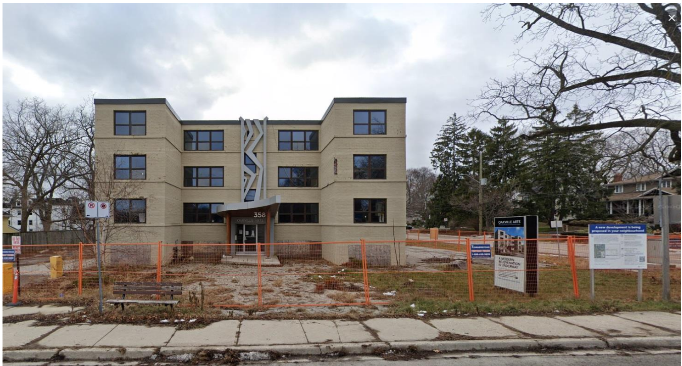
4.1.5.1.A - Existing Northeast (Front) Elevation
