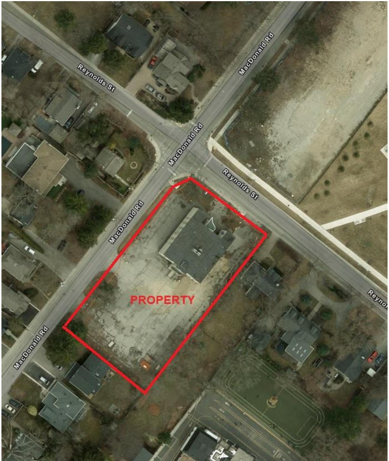
4.1.1.B - Aerial Photograph – Property
