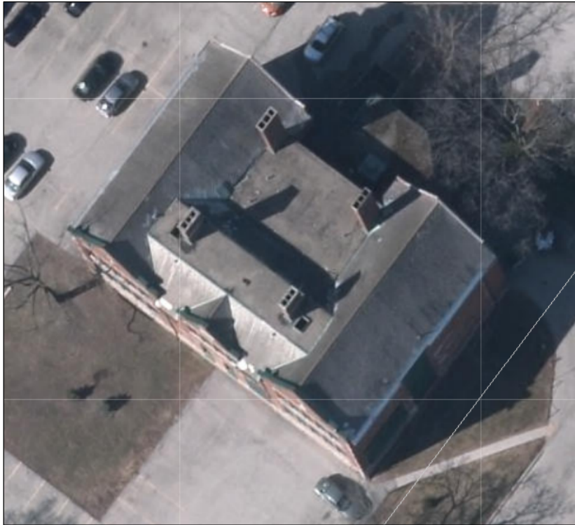
Left: A bird's eye view of the chimneys at 291 Reynolds Street (Source: Town of Oakville, GIS)
