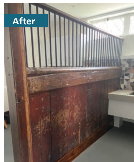
Left: Historic horse stalls after the removal of 1997 materials, 2021; Right: Horse stall partitions retained and incorporated into a new kitchenette, 2022.
