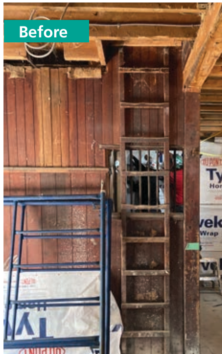
Left: Original hay loft ladder and hatch after removal of 1997 materials, 2021; Right: Ladder and faux hatch after restoration, 2022.
