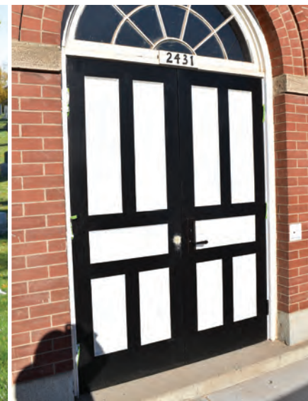
Palermo Schoolhouse with new wood doors installed in 2016
